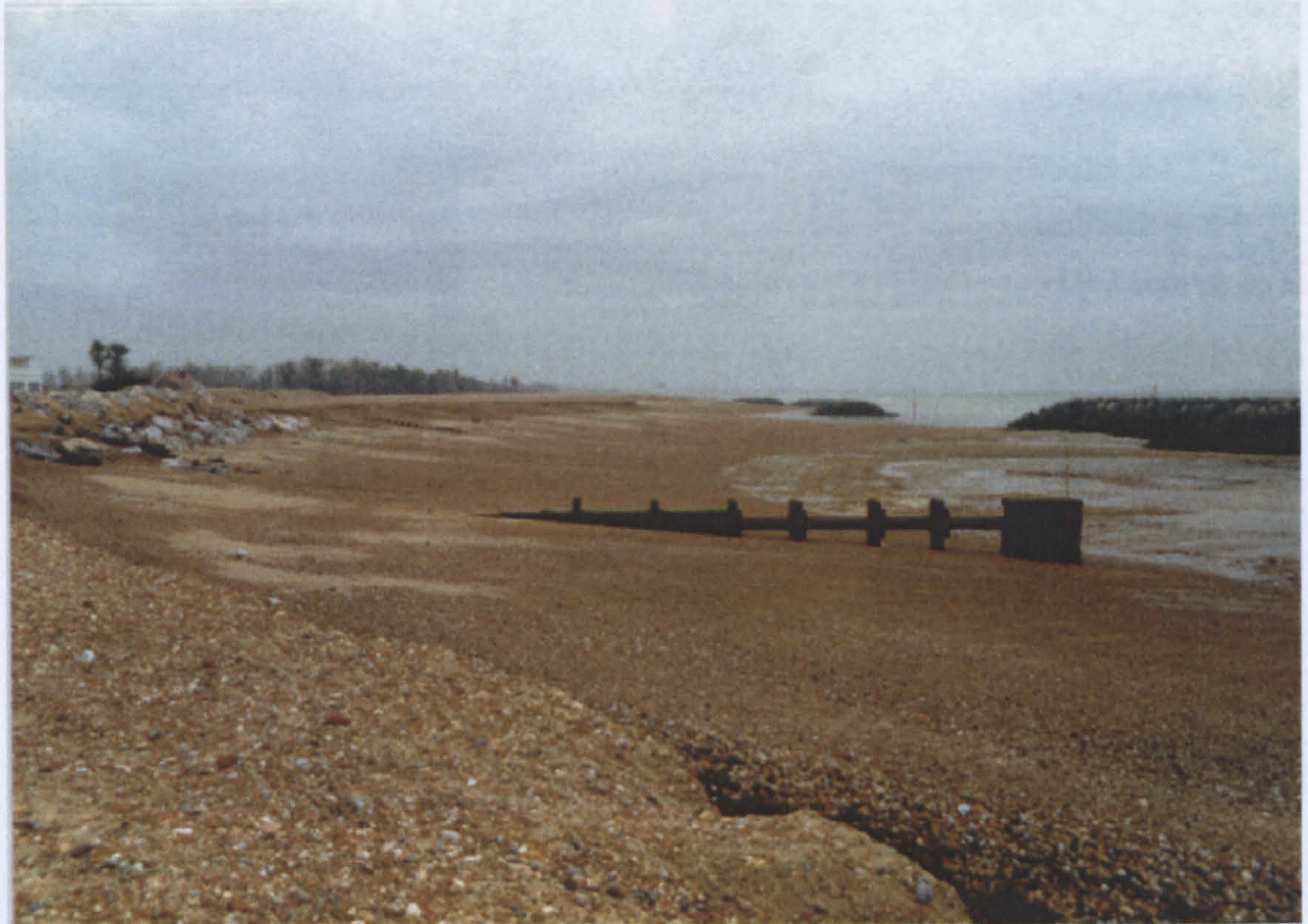
Figure 4-11 Bay 5 revetment (low tide) February 1994. Photograph by the author
