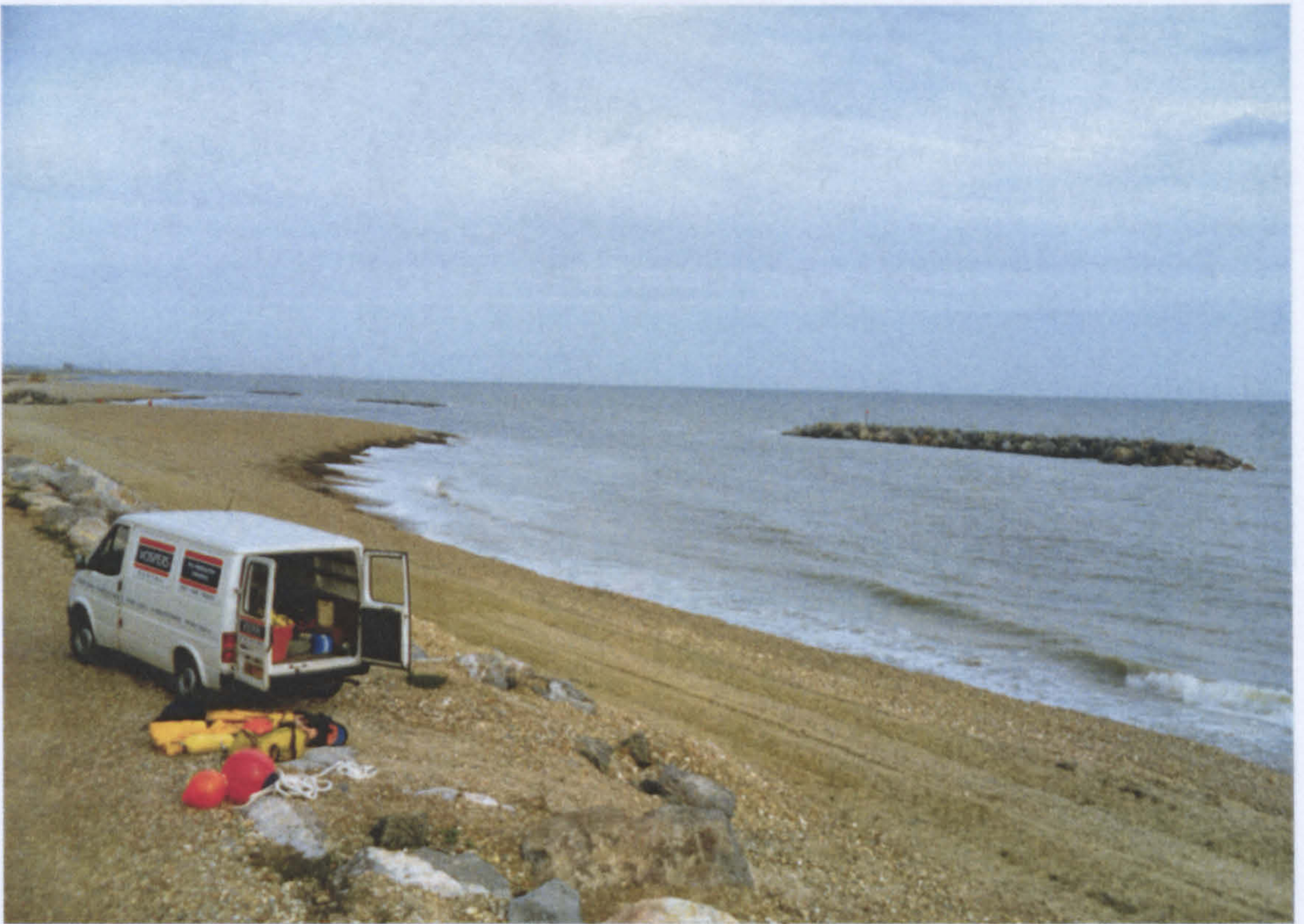
Figure 4-10 Beach in front of bay 5 revetment, High water, September 1993. Photograph by the author
