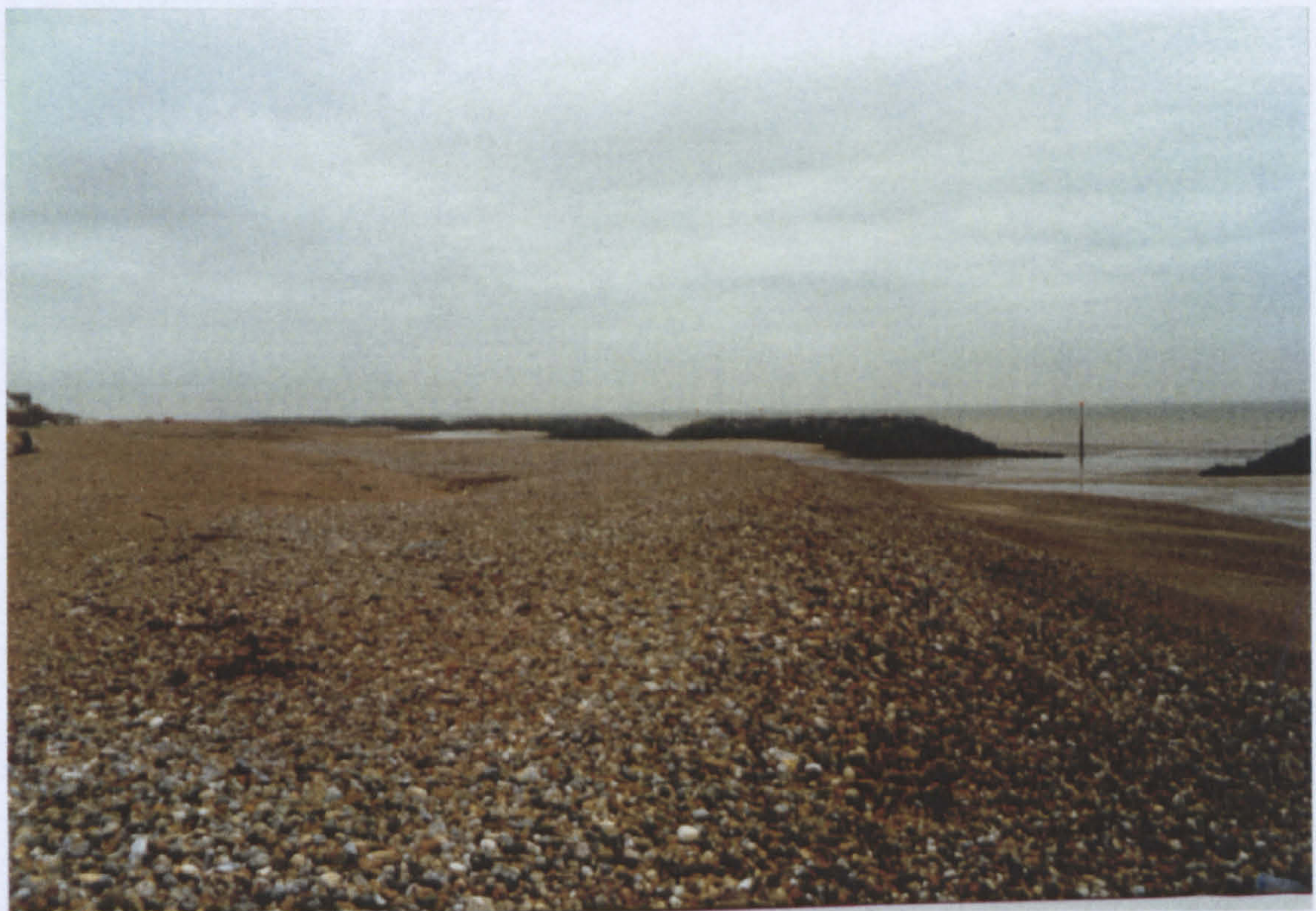
Figure 4-9 Shingle accretion behind breakwater 1 (photograph by the author)
