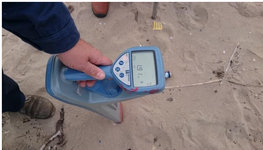
Figure 25 RD receiver during locating existing lines before cable landing works in Italy (courtesy Subsea Cable Tracking Ltd)
