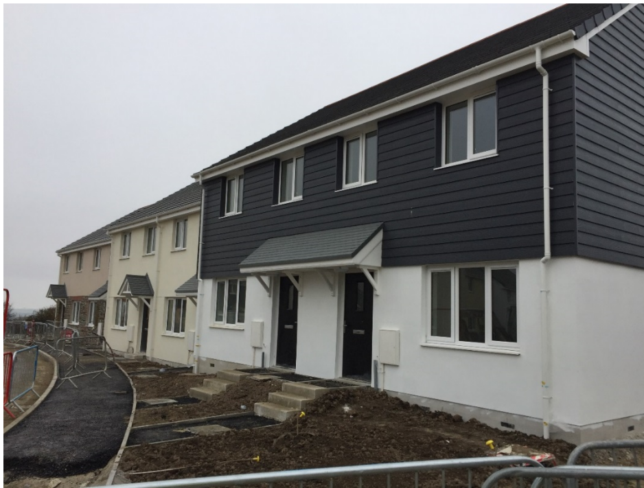
Figure 3-7 Case study 1 general view (Source: Taken by this thesis' author)
