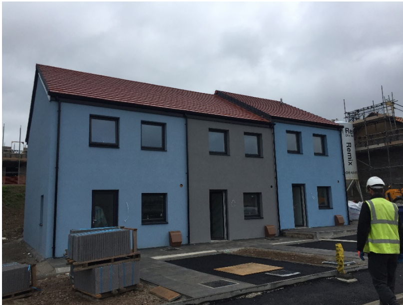
Figure 3-13 Case study 4 general view (Source: Taken by this thesis' author)
