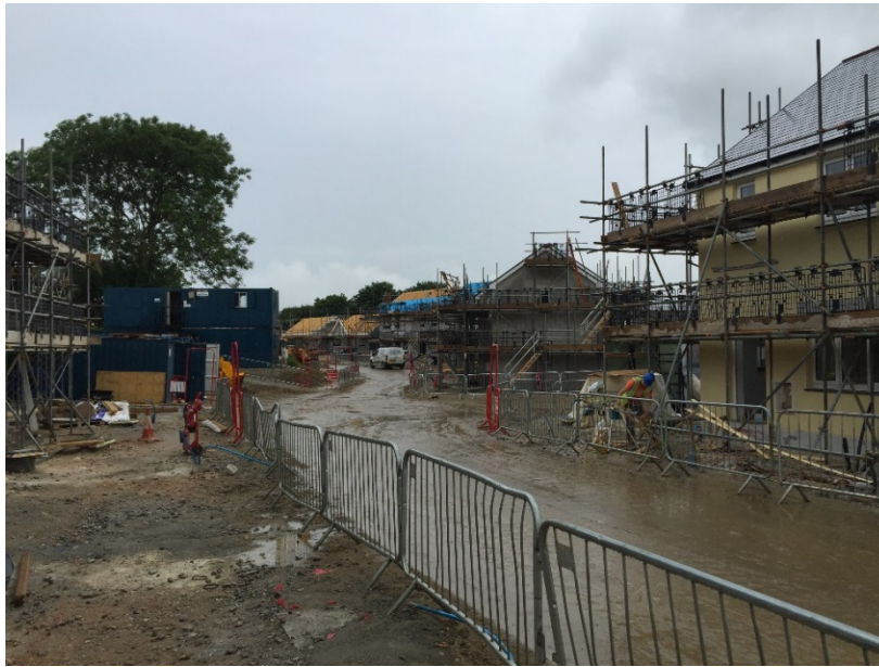
Figure 3-9 Case study 2 general view (Source: Taken by this thesis' author)
