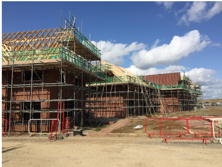
Figure 3-15 Case study 5 general view (Source: Taken by this thesis' author)
