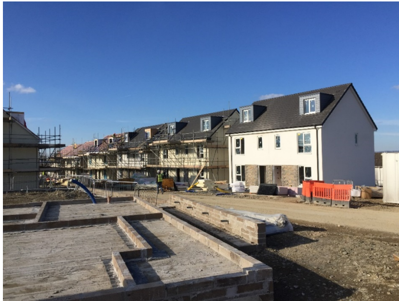
Figure 3-11 Case study 3 general view (Source: Taken by this thesis' author)
