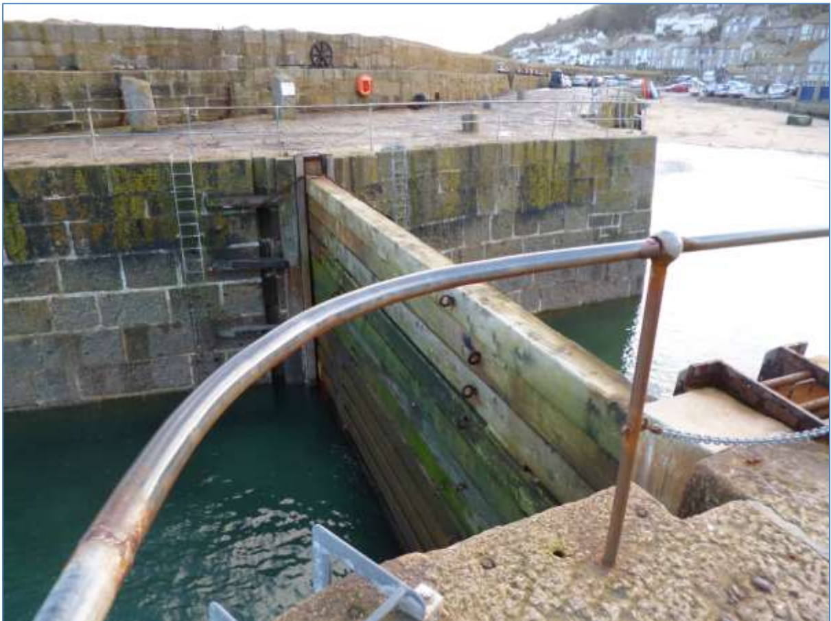
Figure 5-5 : The port of Mousehole harbour entrance : wooden baulks - Source : ( Author )
