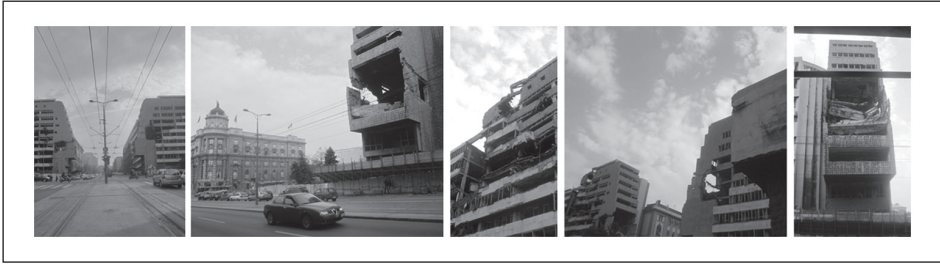
Figure 2. The Generalstab complex in (w)hole after 1999.
