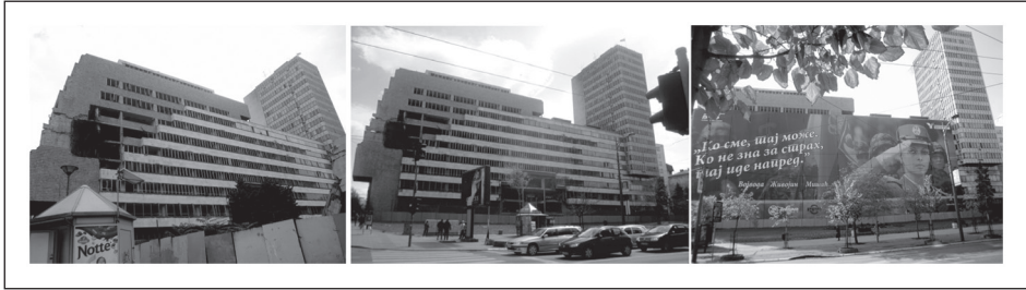
Figure 3. The Ministry of Defence – building ‘B’ in 2010, with the entry foyer removed and replaced with the billboard in 2015.
