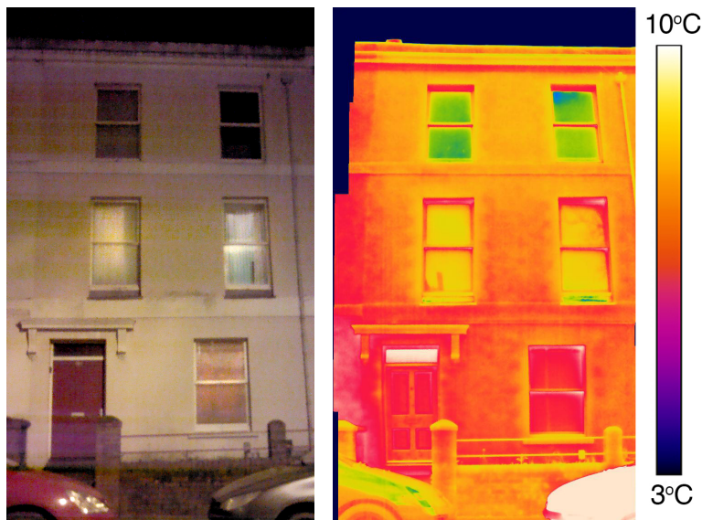
Figure 14. Photograph showing dwelling lighting to help indicating occupancy during analysis of thermal image.
