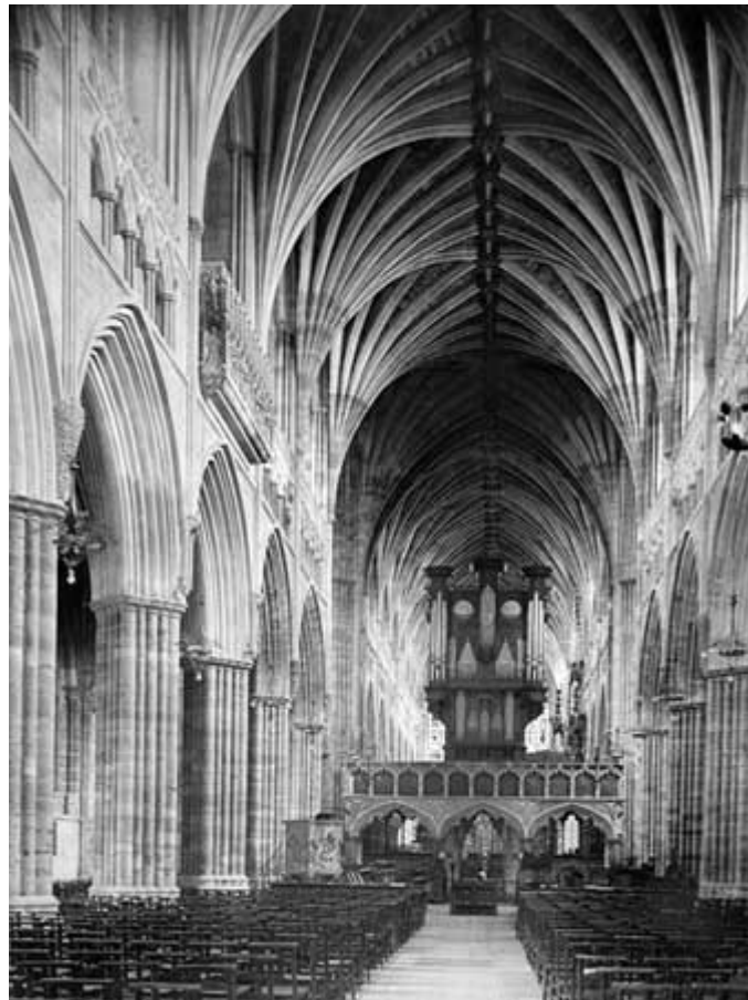
Figure 11: Interior of Exeter Cathedral: Nave looking East., Exeter Cathedral Archive; [Photographs not catalogued at the time of consultation]
