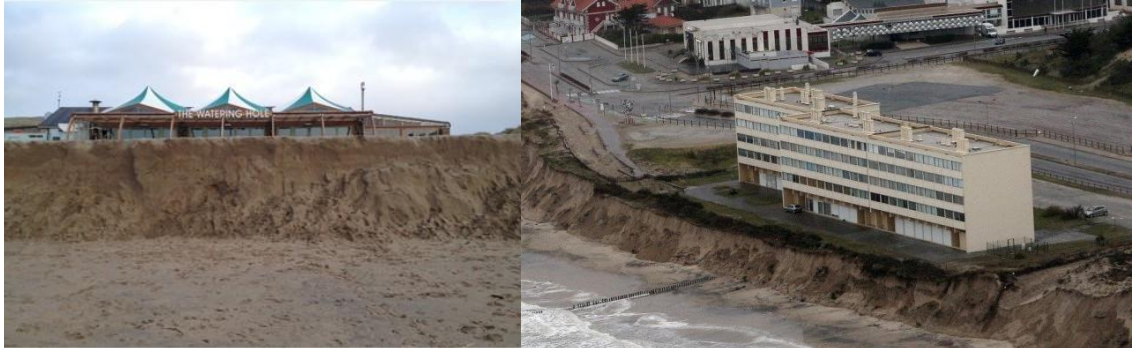
Figure 10.1 Consequences of 13/14 winter storms at Perranporth Beach (UK) and Soulac-sur-Mer (France) on the left and right hand, respectively
