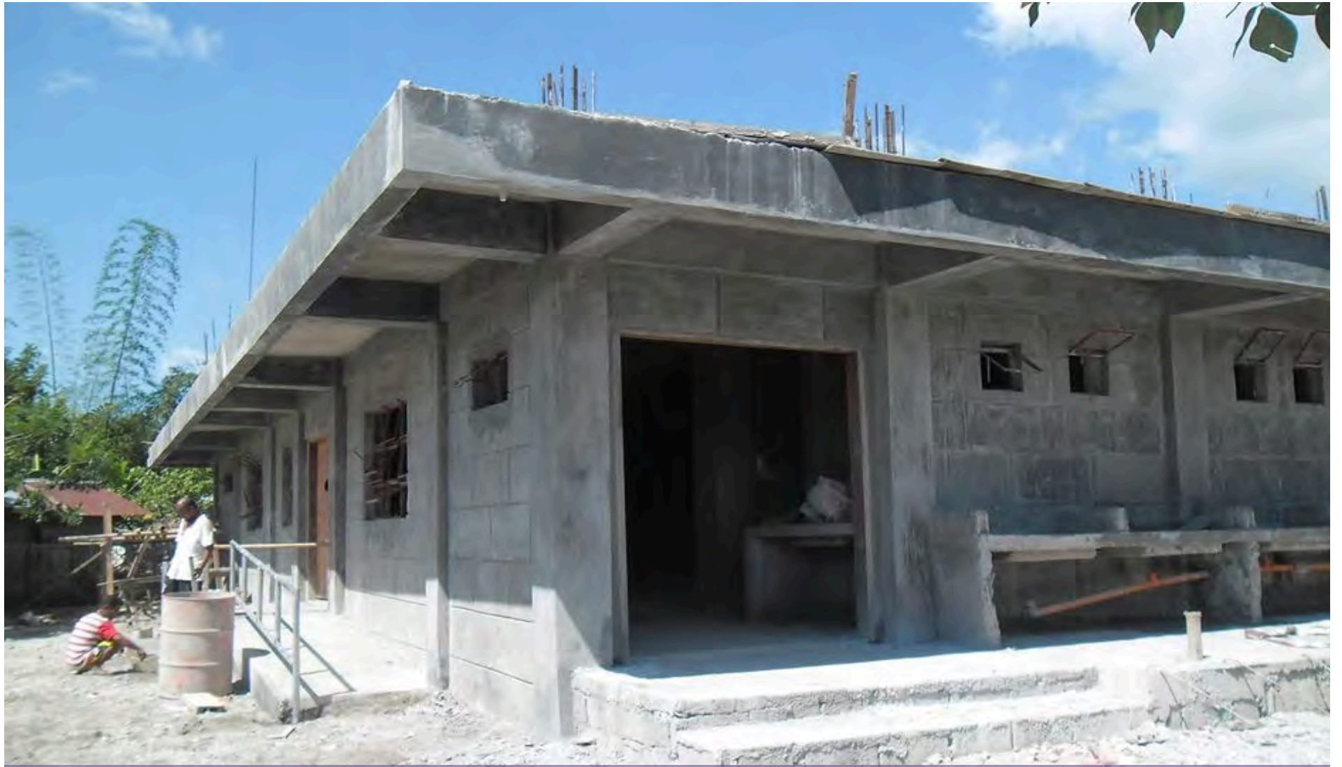
Community Co-Designed and Managed Evacuation Center
