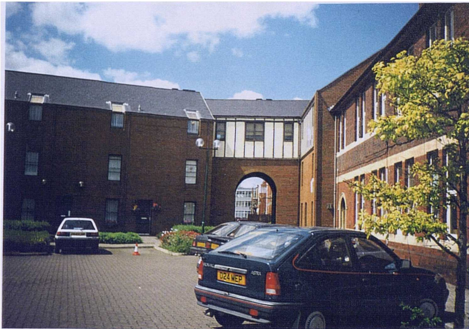
Figure 4.19 View into Pier Street from East Burrows Road
