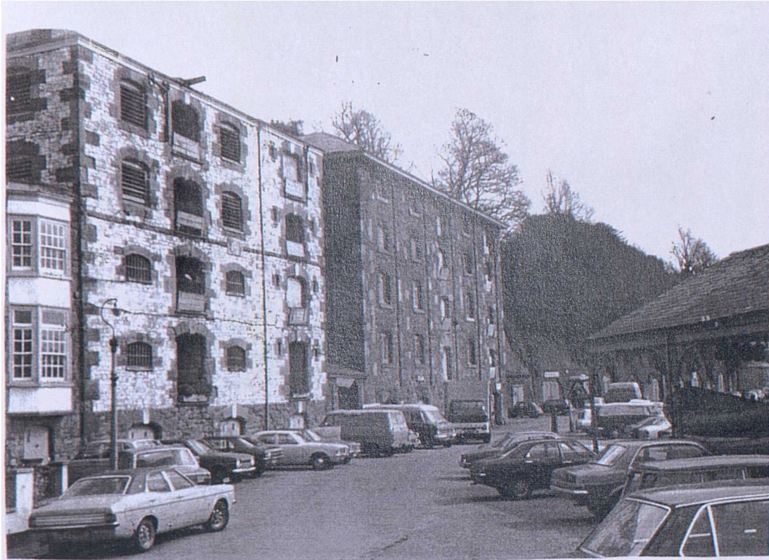
Figure 4.2 Quay area prior to regeneration
