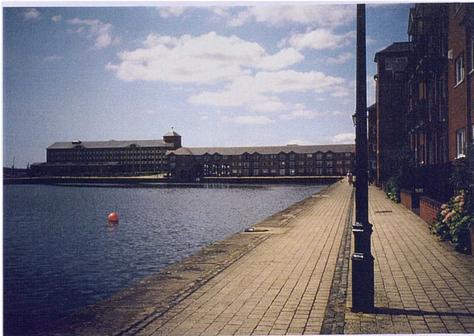
Figure 3.9 Walkway at Swansea Maritime Village
