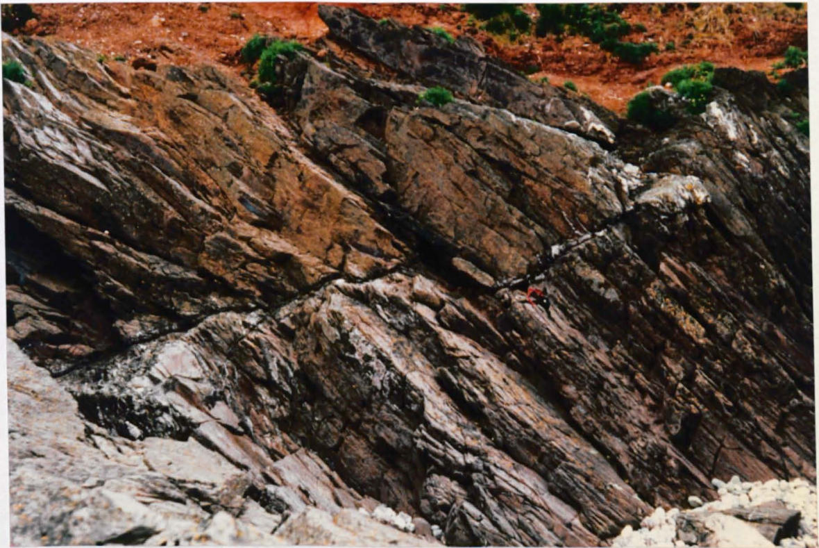
Plate 4.44 Extensional fault displacing a Variscan thrust. Fault forms parallel to and re-activates the first phase Variscan cleavage; Westlake Bay [SX 4925 4920]. Looking north east.
