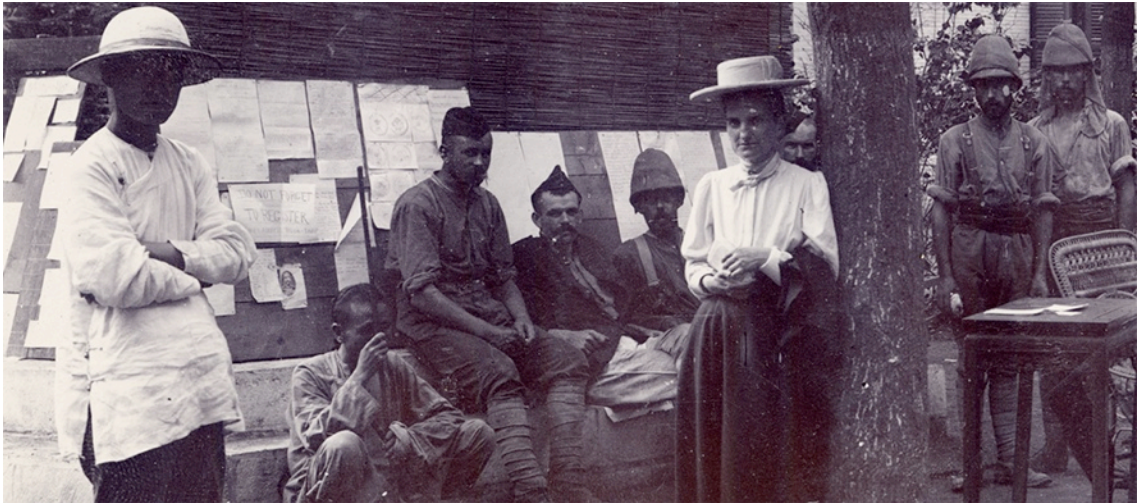
Figure 134. Detail from the “Bell Tower.”
