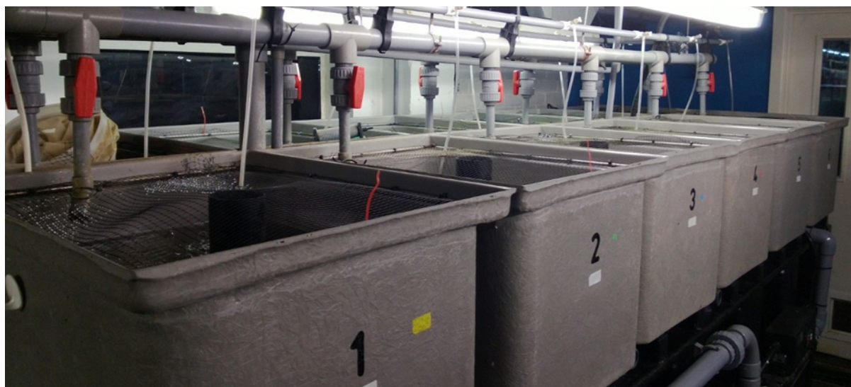
Figure 3.5: Sideview of recirculation system of Aquatic Animal Nutrition and Health Research Group Aquarium, University of Plymouth
