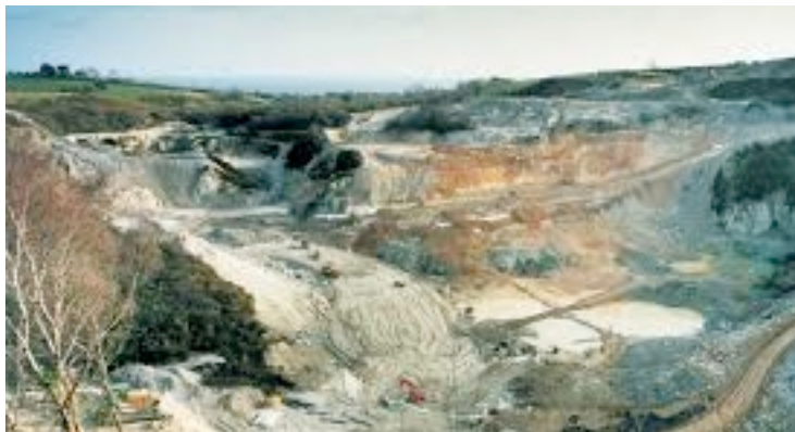
Figure 7 The clay mine before start of construction, Cornwall 1995. Photo the Eden Project
