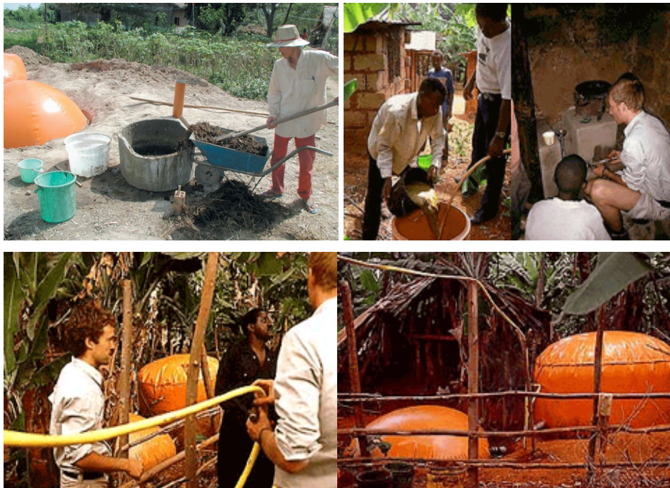
Figure 1 Installing the Supergas bio-reactor in Tanzania 1997 (all Photos Superflex)
