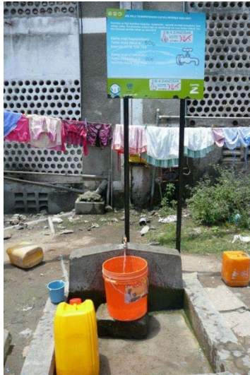
Figure 12 Well with billboard showing well code number and SMS number for water collectors to send information to. Photo HSW 2009 ( www.h20initiative.org )
