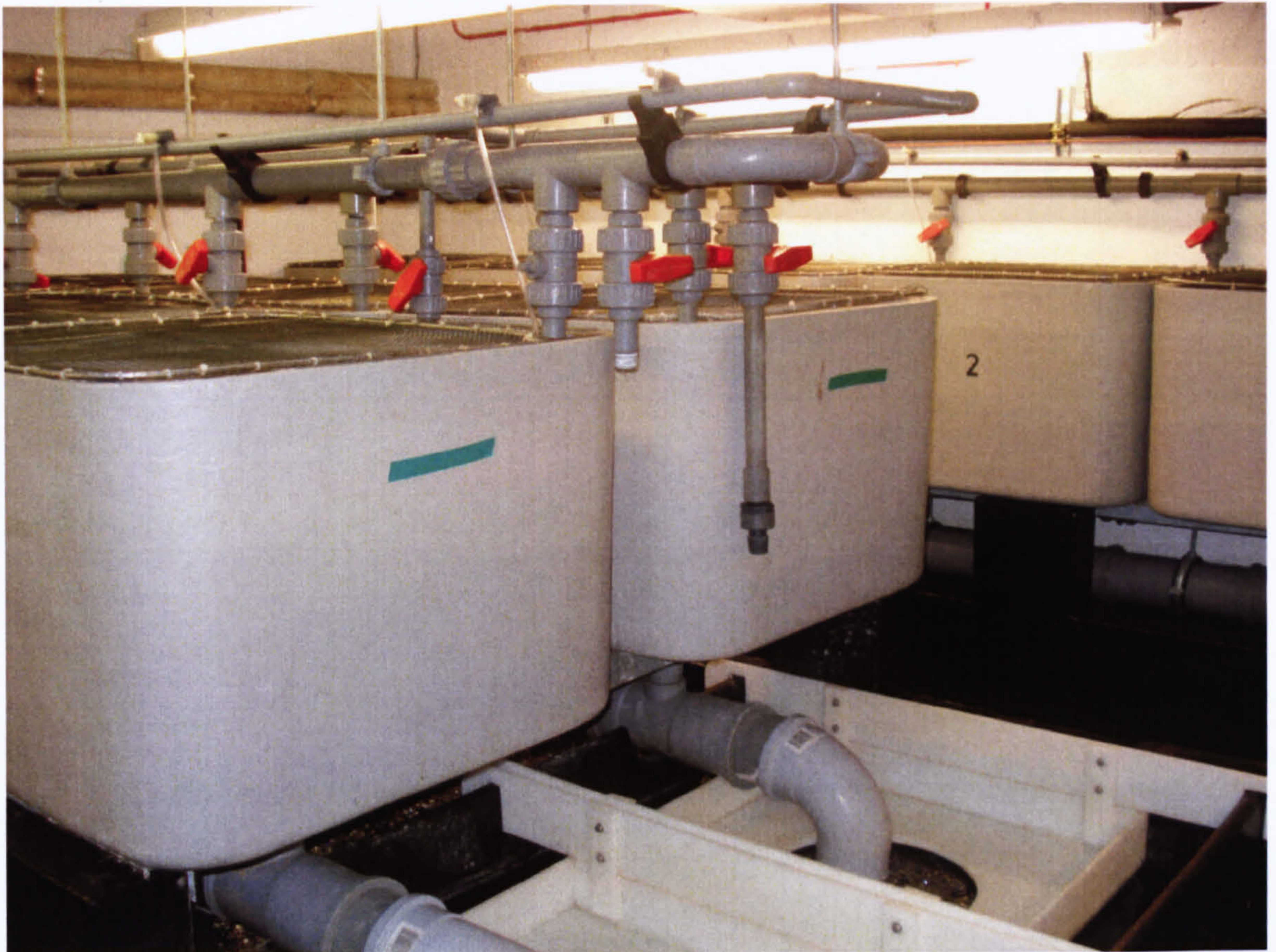
Plate 3.3. Recirculation system A, Aquaculture and Fish Nutrition Research Aquarium, The University of Plymouth.
