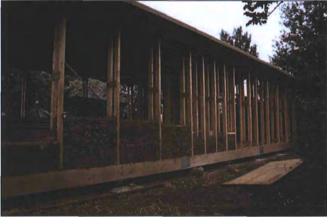
Figure 27: The clay straw studio under construction
