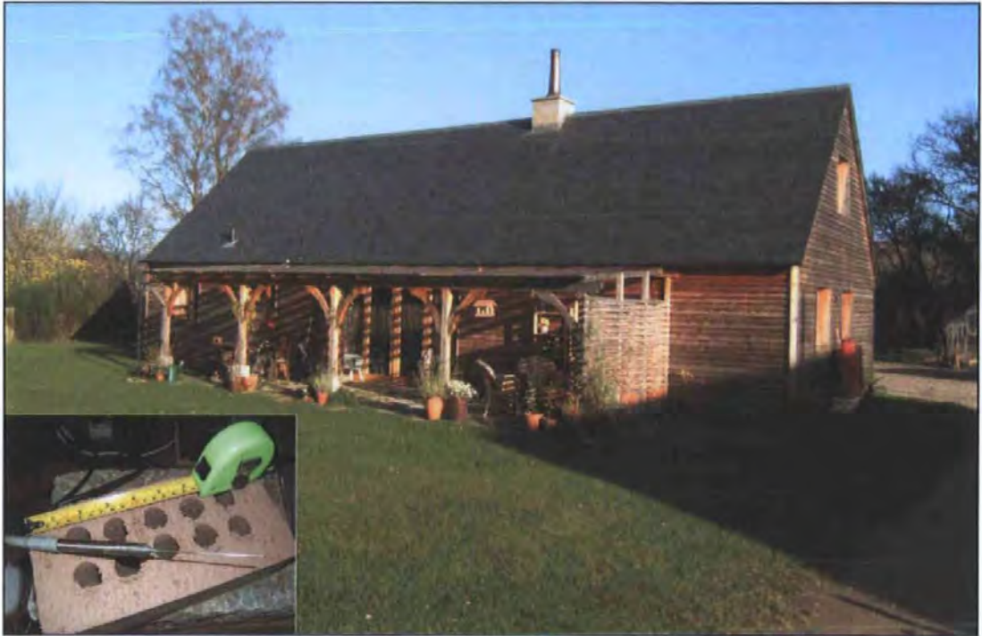
Figure 23: Unfired earth and woodshaving brick house with an example brick
