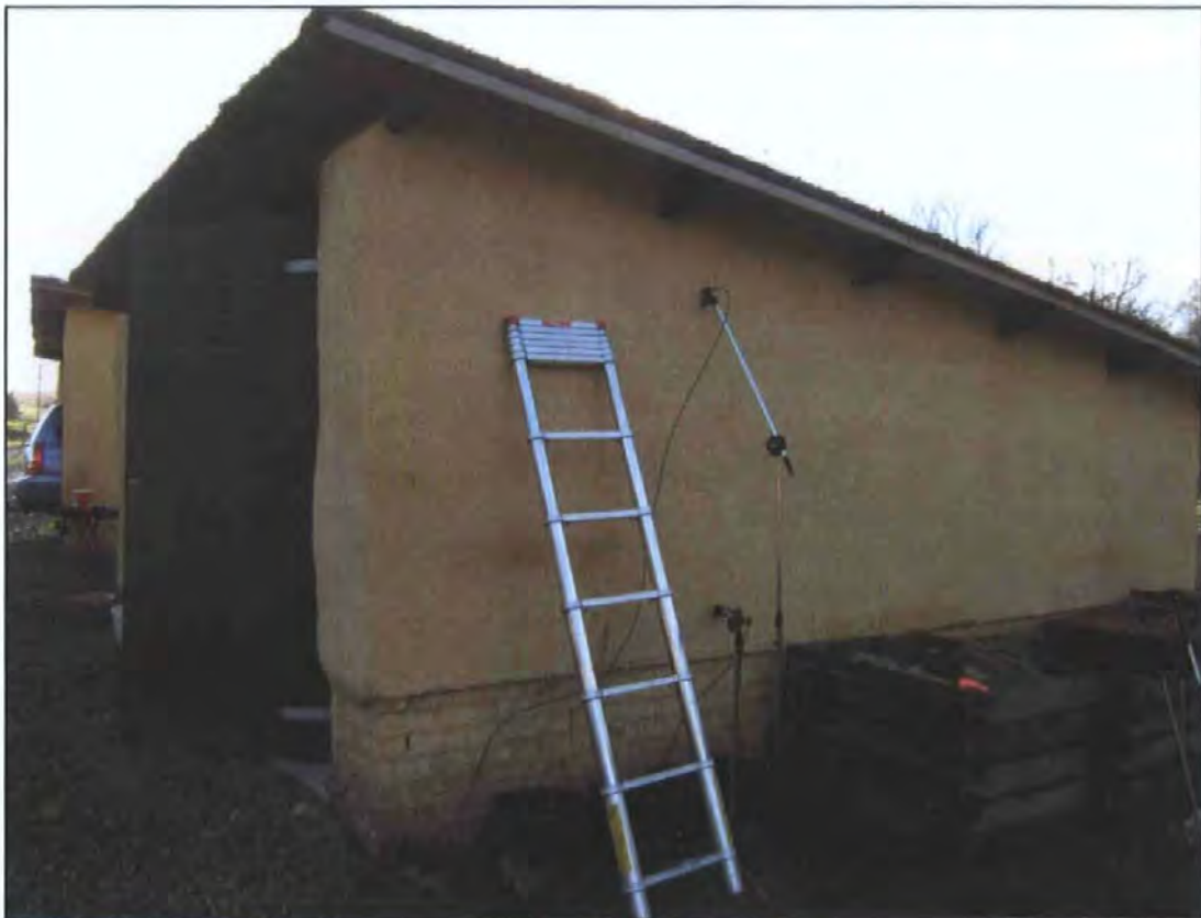
Figure 24: Straw bale garages with probes in situ
