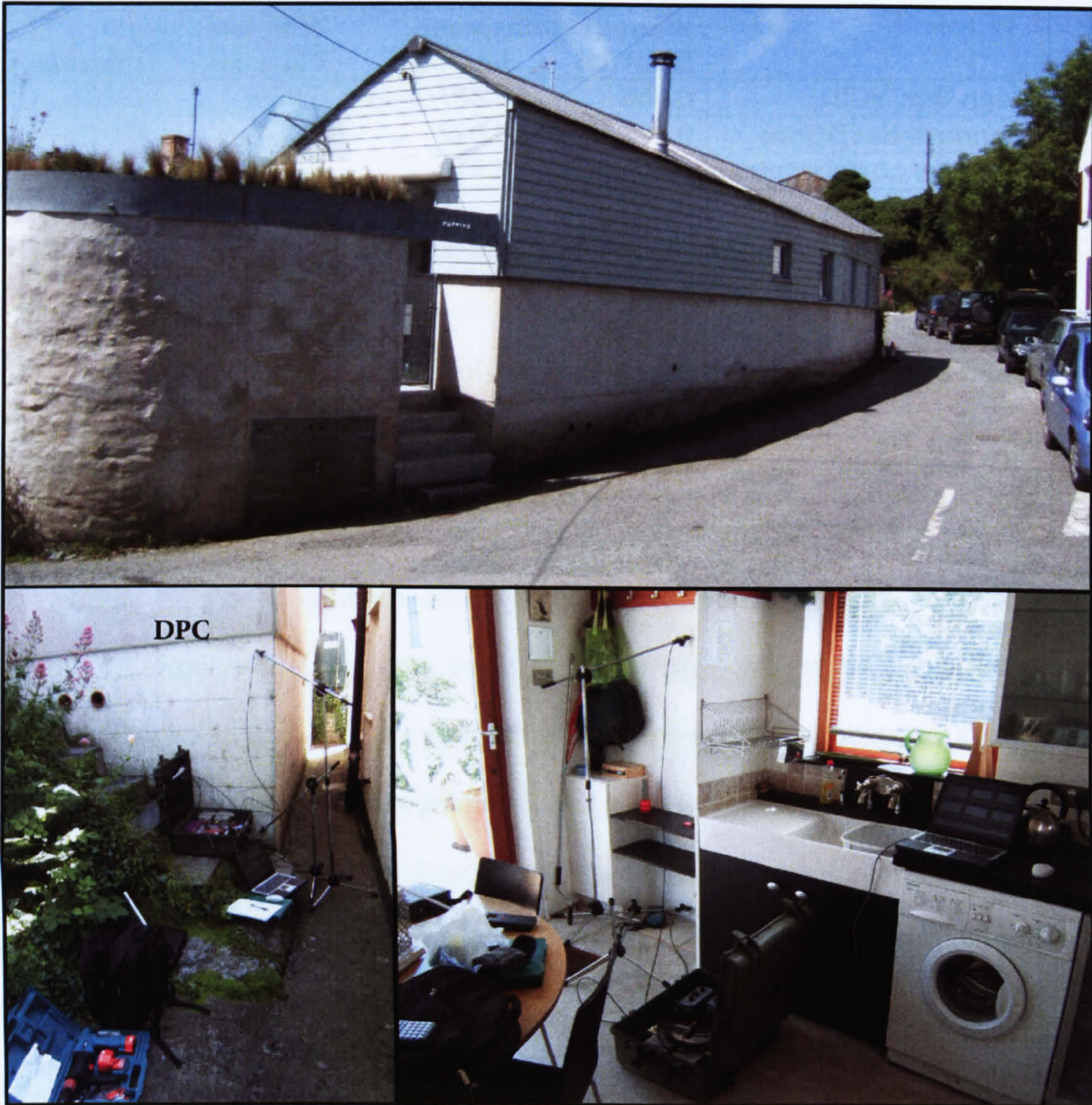
Figure 22: North Cornwall eco-house showing various measurement positions
