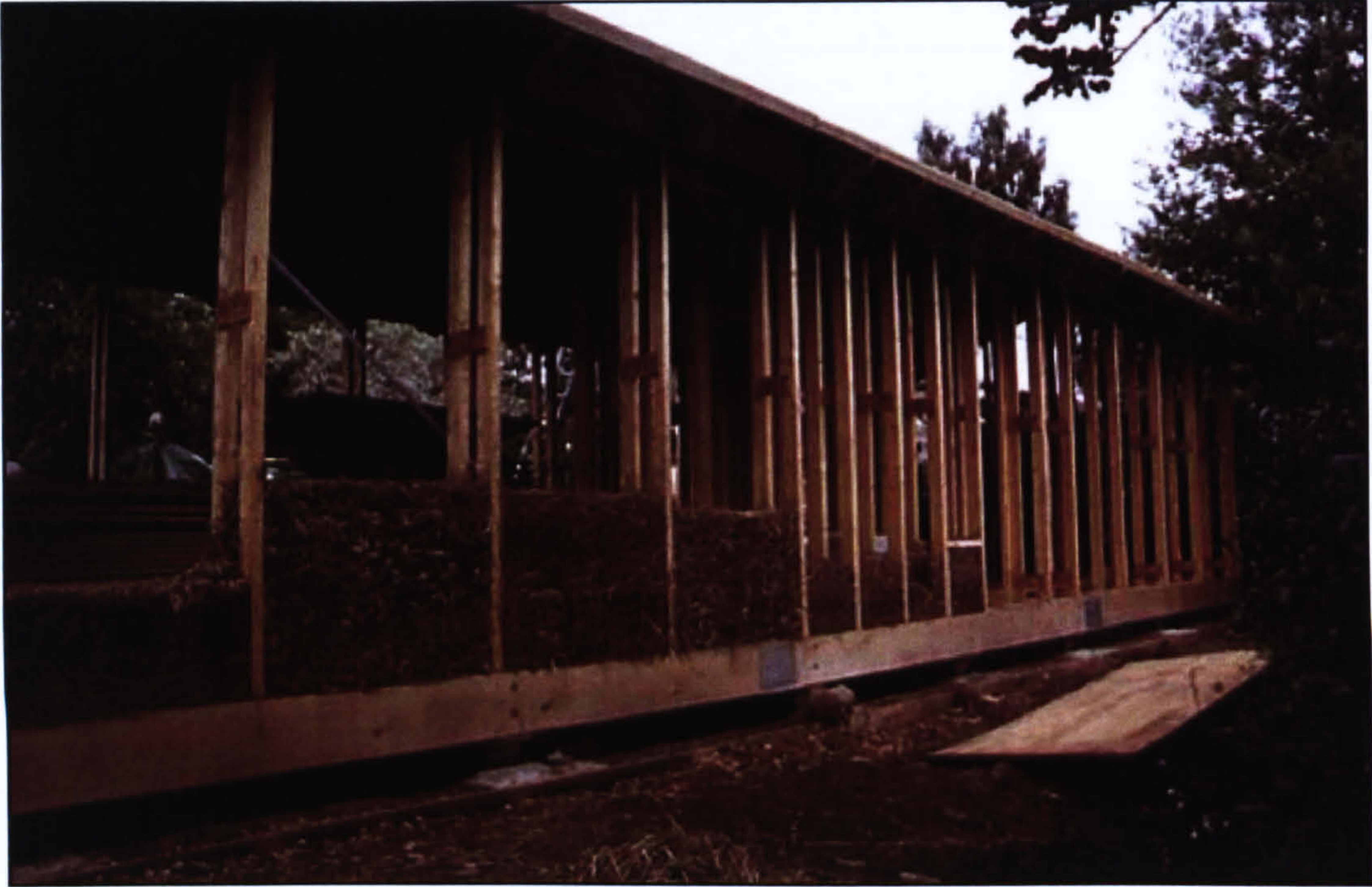
Figure 27: The clay straw studio under construction
