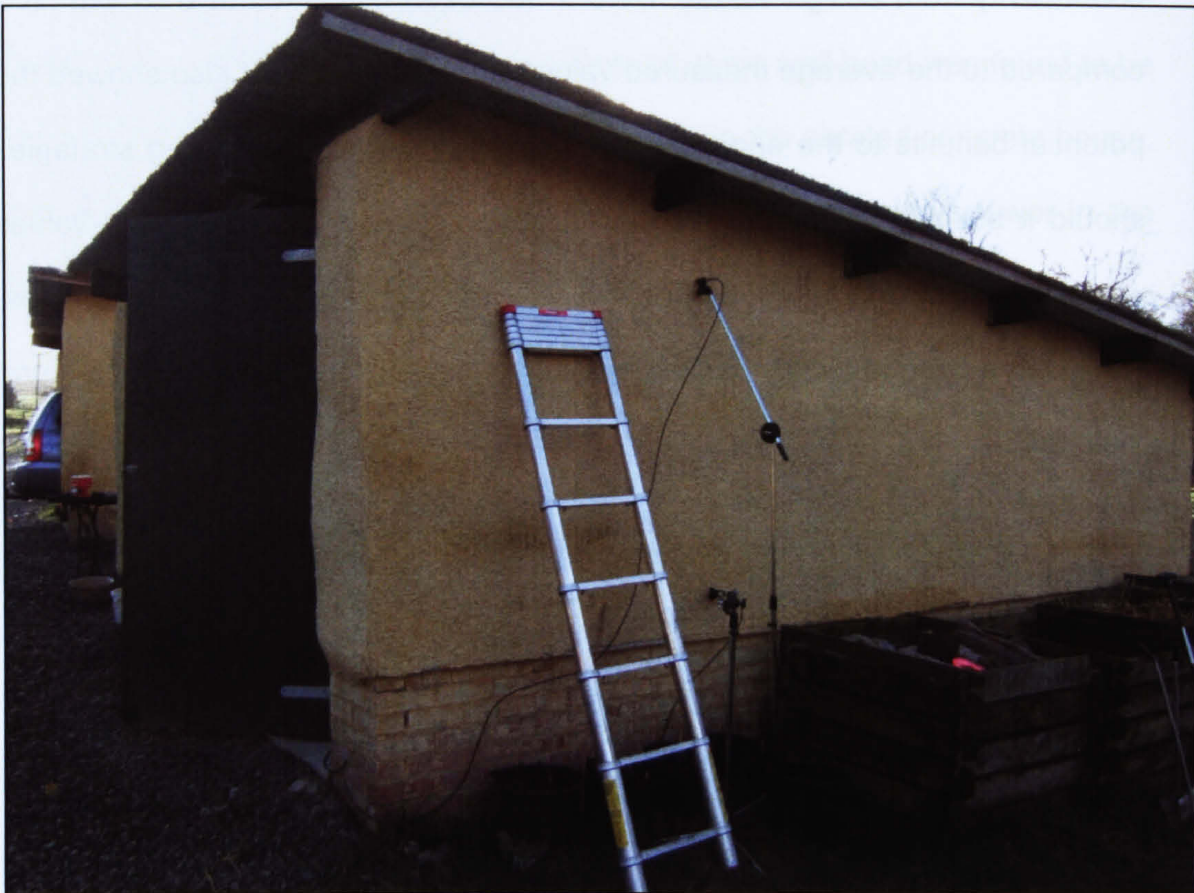
Figure 24: Straw bale garages with probes in situ
