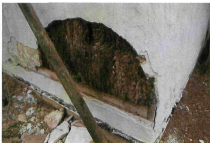
Fig.97 Corner of a wall at Cuckoo farm, where the render has failed.
