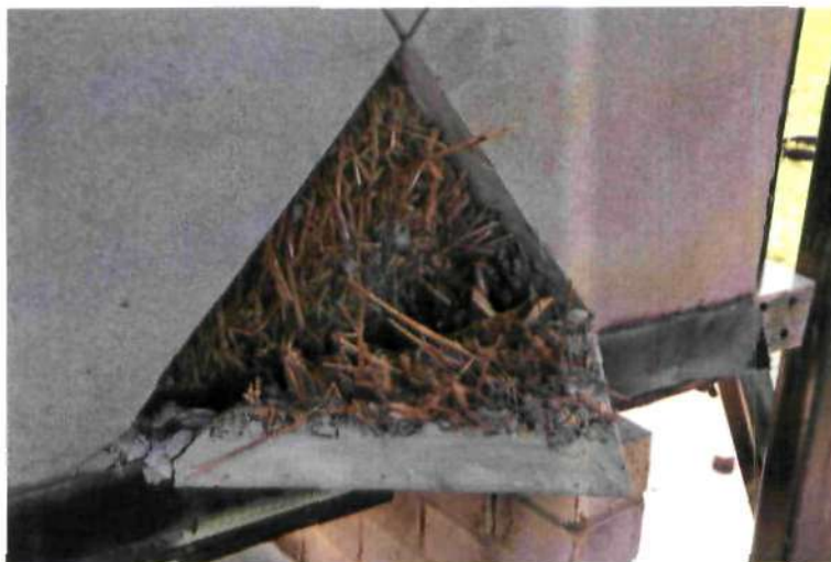
Fig.A11 Section of render removed from panel
