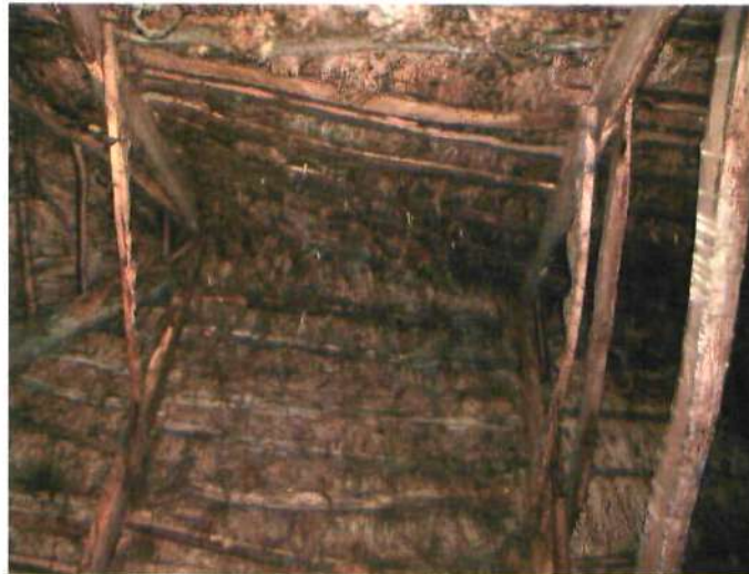
Fig.4 Five hundred year old smoke blacked thatch at Uppacott
