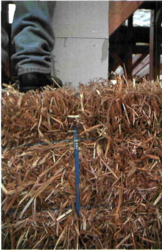
Fig.66 Bale laid on edge, held against post with polypropylene strapping.
