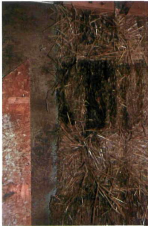
Fig.A23 Water damage at Atkinson Cottage
