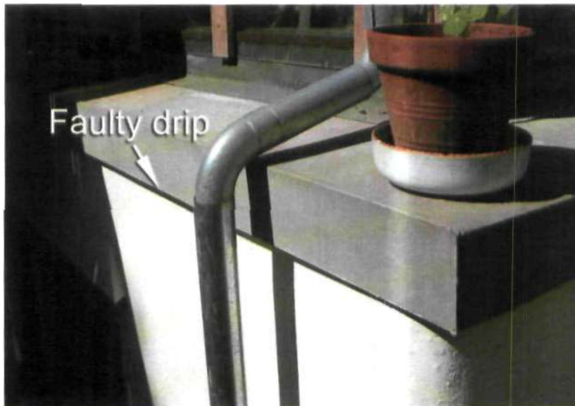
Fig.71 Location of faulty drip detail above bedroom 1
