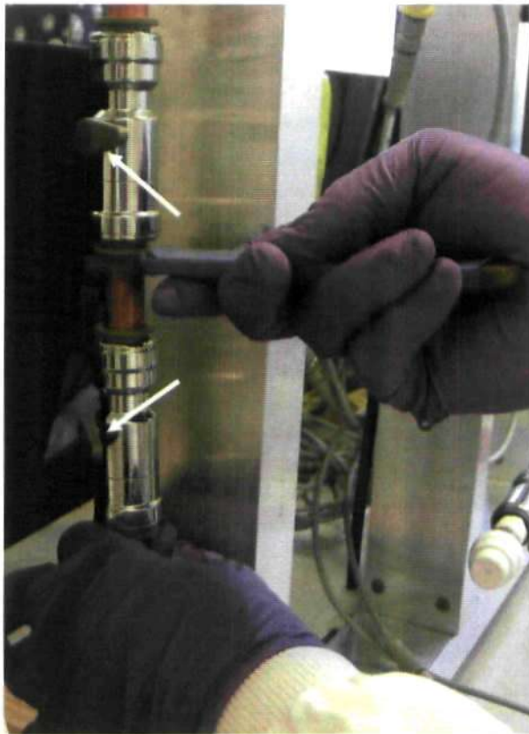
Figure 2.7 Removal of copper insert from test rig system. The chrome ball valves above and below the insert of interest are in the 'closed' position, as indicated by white arrows.
