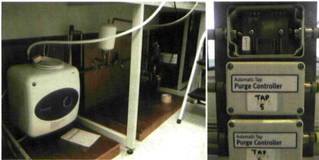
Figure 2.4 Detail of services supplying test rig, including (left) heater and storage tank, and (right) automatic tap purge controller.
