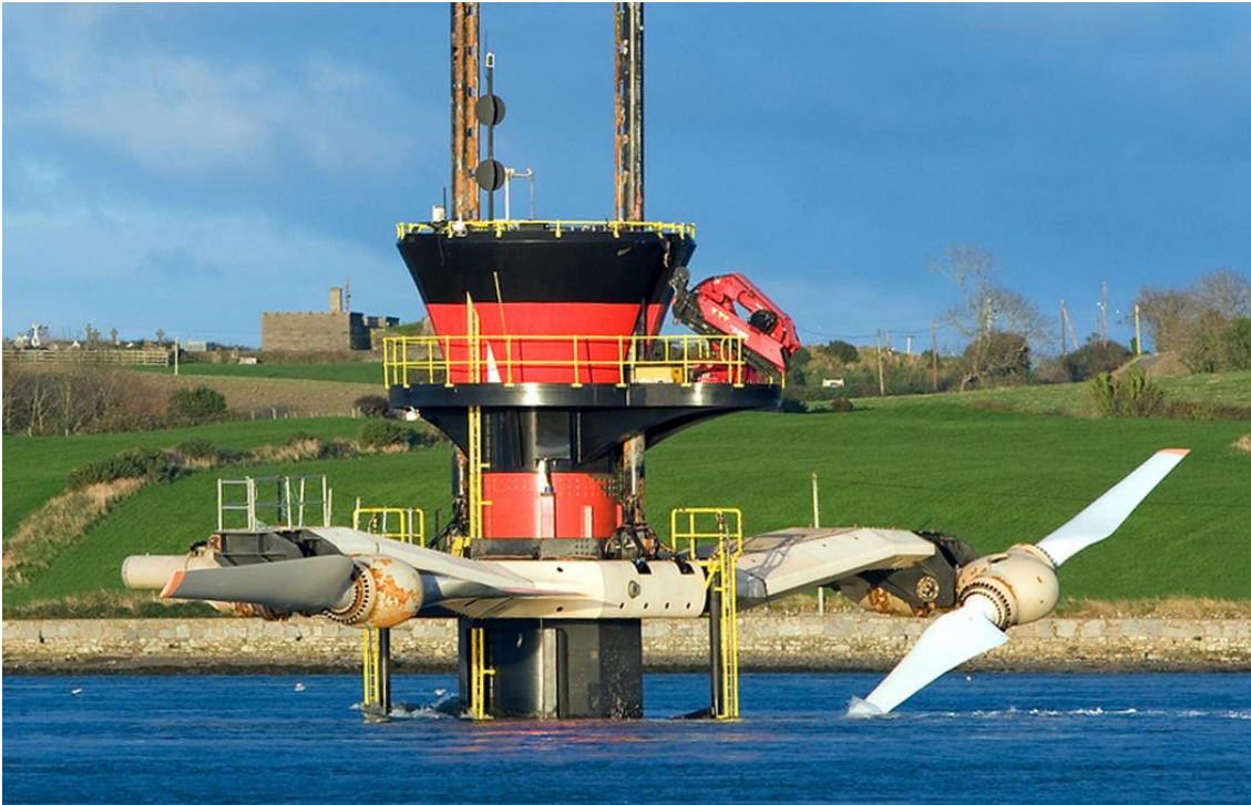
Figure 1.1 The 600-kW marine current turbine installed in Strangford Lough in County Down, Northern Ireland (SIEMENS, 2008)
