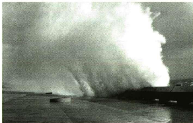
Figure 1.1.5 Severe wave overtopping at Samphire Hoe sea wall (photo courtesy of WCCP/Eurotunnel Developments Ltd)
