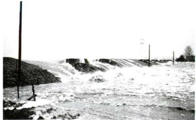
Figure 1.1.4 the failure of a sea dike due to wave overtopping (photo: Zitscher, 1976)
