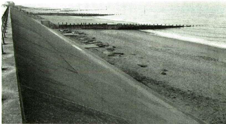
Figure 2.3.4 Hornsea's seawall along the Holderness coast, UK (Source: http://picasaweb.google.com/lh/photo/YCUHTs8PXbwdasEuIh9NRg ).
