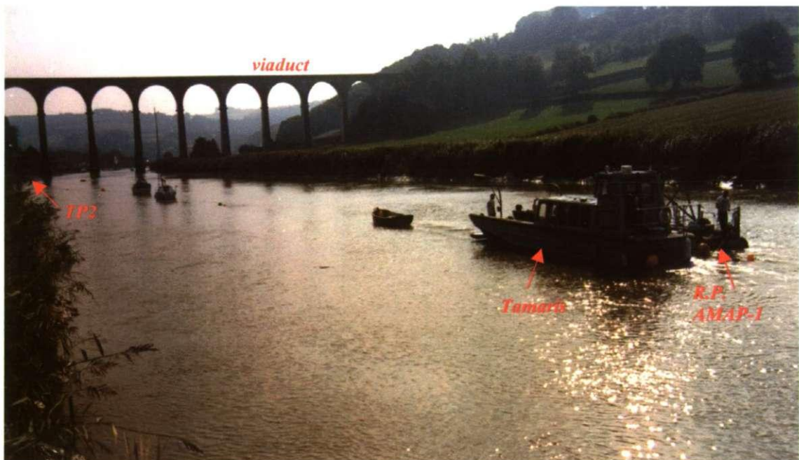
Plate 3.1 Calstock Station A location, looking east towards the viaduct (upstream).
