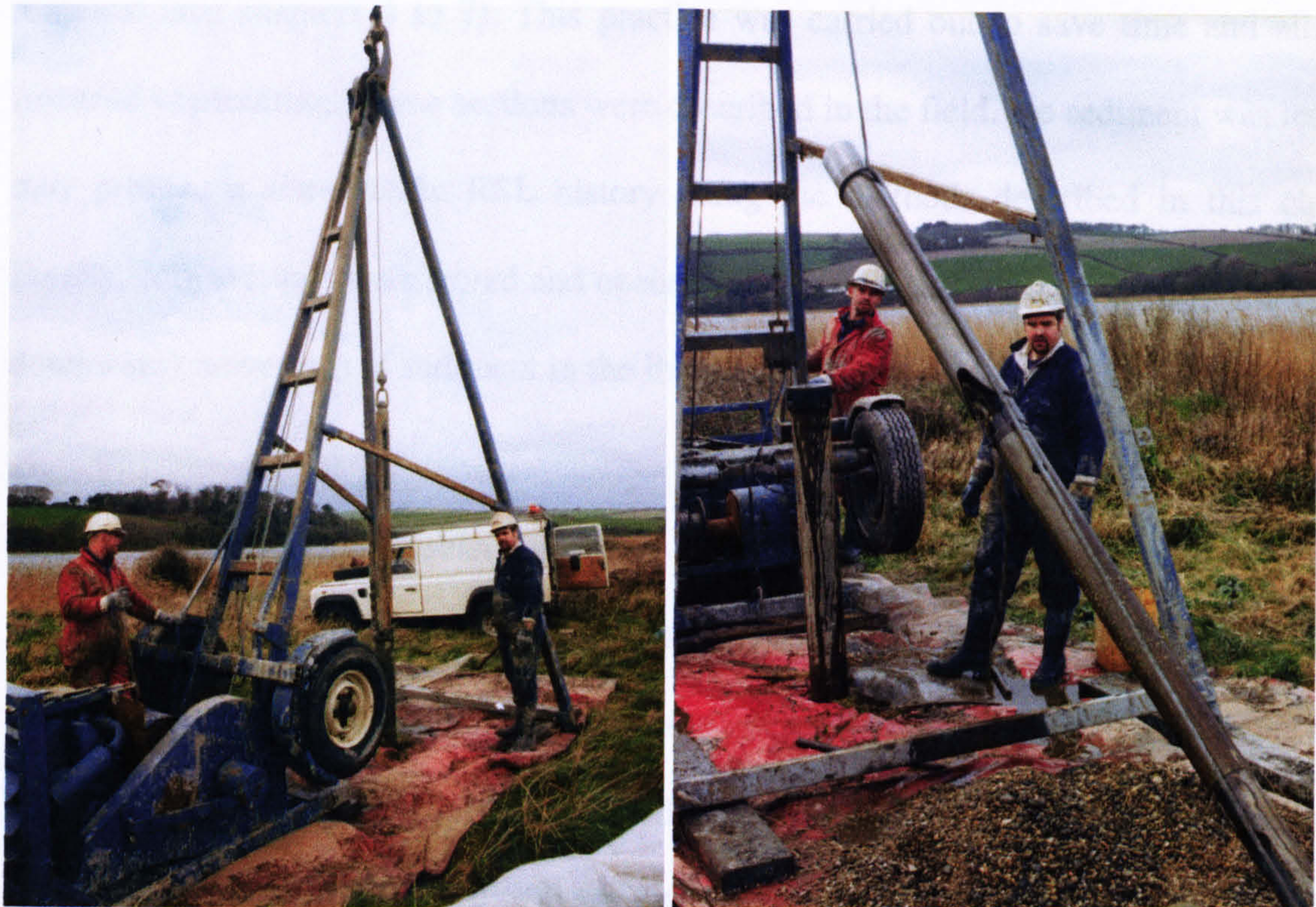
A. Core drilling
