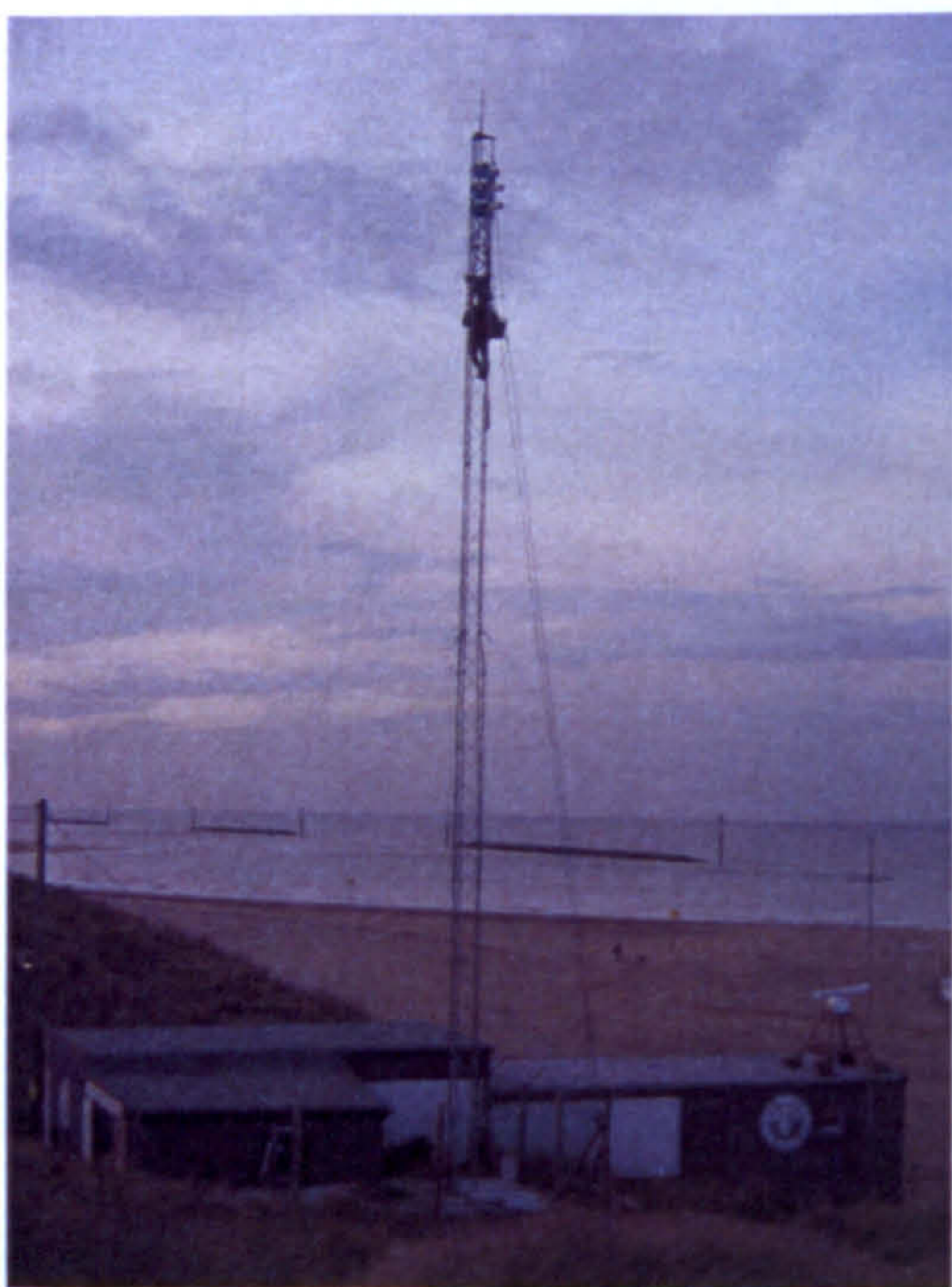
Figure 4.2.3: A photo of the Sea Palling camera tower with guys attached
