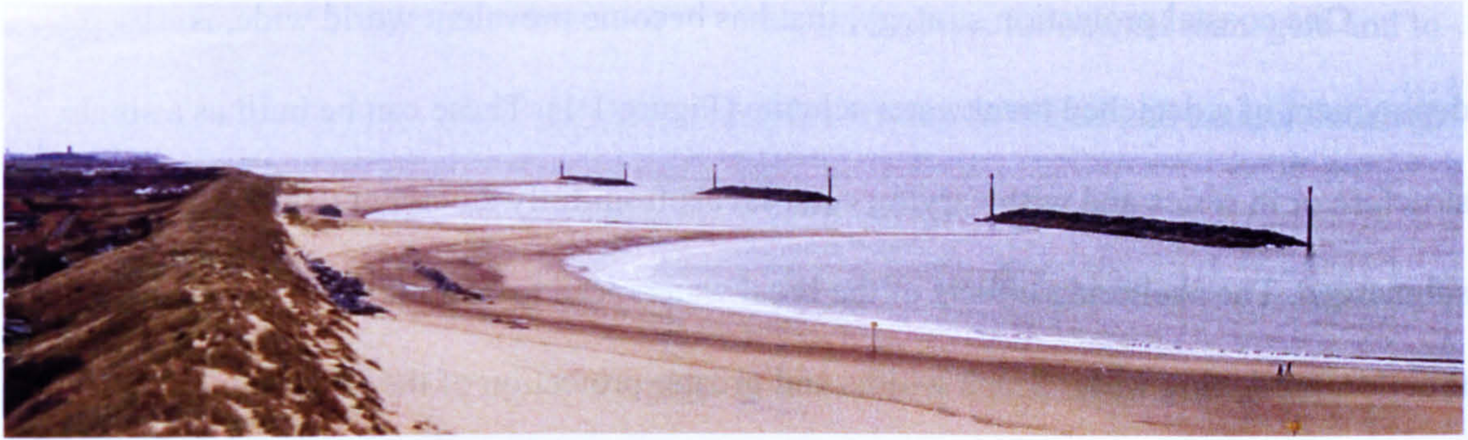
Figure 1.1: A photograph showing three rubble mound detached breakwaters used to protect a vulnerable village. The accumulation of sediment behind the breakwaters, in the form of tombolos, can clearly be seen. Also observable is the formation of an embayed beach between the two structures.
