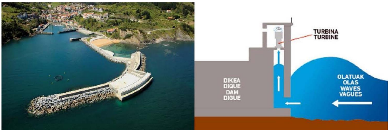
Figure 12: Mutriku's breakwater-mounted OWC (left) and schematic of the system (courtesy of EVE [92])
