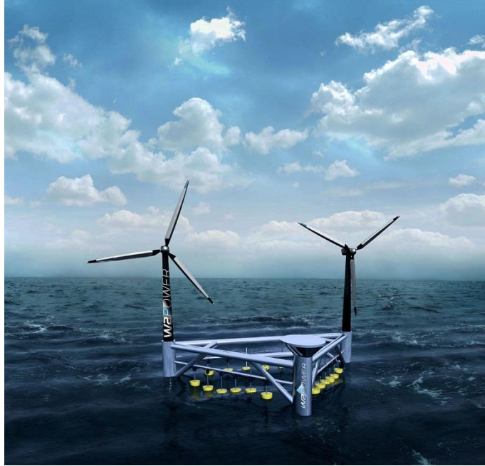
Figure 6: Artist's impression of a floating hybrid system W2Power (courtesy of Pelagic Power AS [50])
