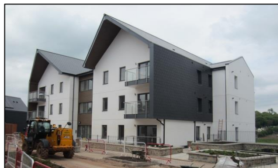
Figure 1 Case study apartment building constructed to Code for Sustainable Homes Level 4
