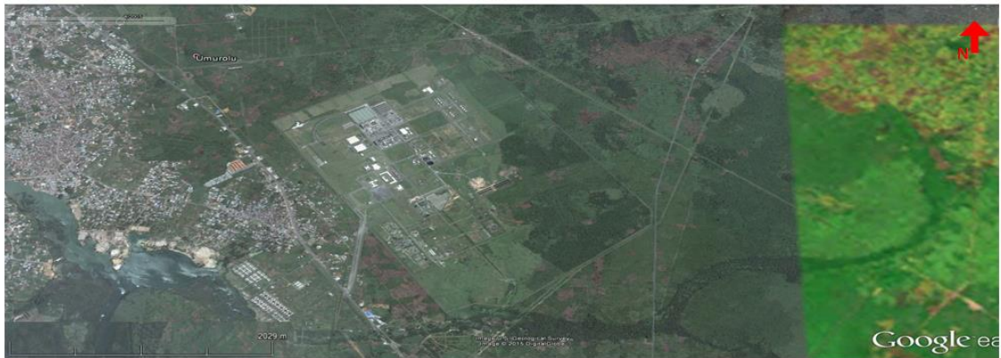
A: Umurolu Flow Station, 2005 (Google Earth)
