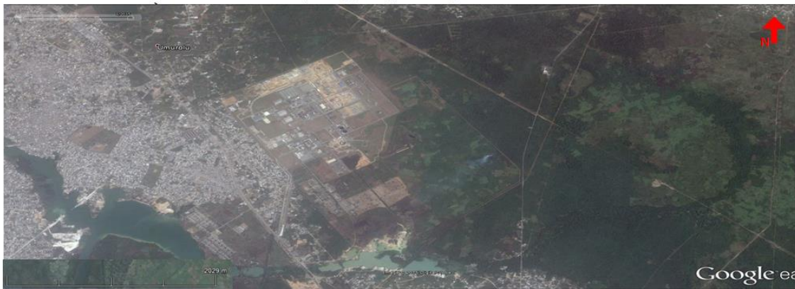
B: Umurolu Flow Station, 2015 (Google Earth, 2015)
