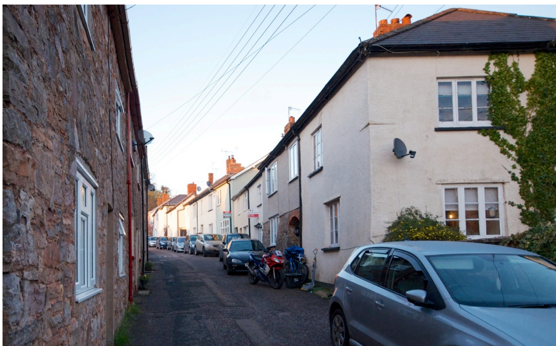
Figure 101. Photograph of case study B street.
