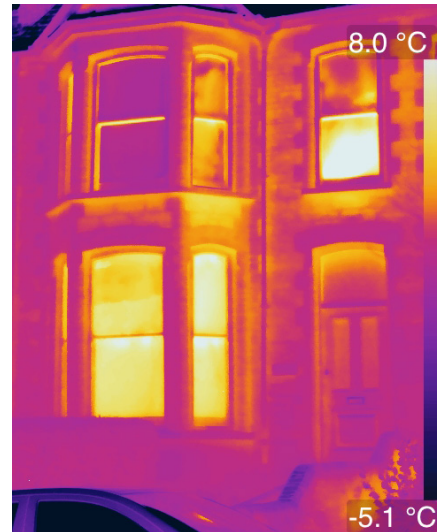
Example street view thermal image
