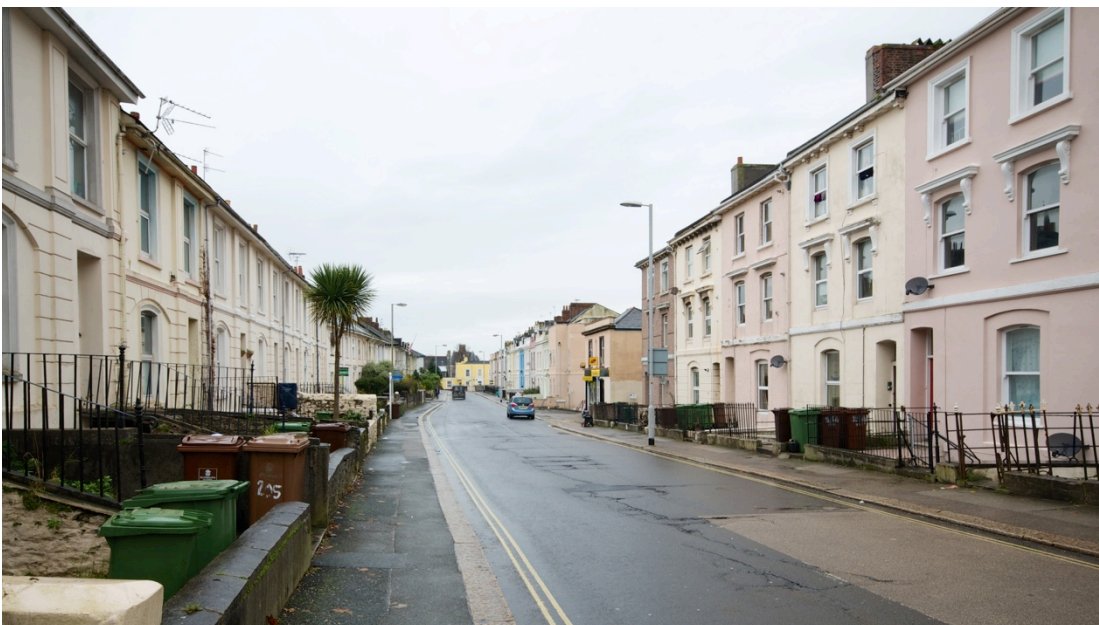
Figure 99. Photograph of case study A street.
