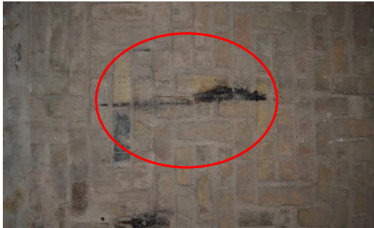
Fig 3.22. The unsuitable walls situations due to lightening candles: a) The soot accumulated due to burning candles beside the wall, b) The soot which has to be cleaned and after 3 years, the appearances of walls are the same
