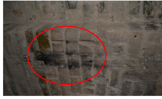
Fig 3.22. The unsuitable walls situations due to lightening candles: a) The soot accumulated due to burning candles beside the wall, b) The soot which has to be cleaned and after 3 years, the appearances of walls are the same
