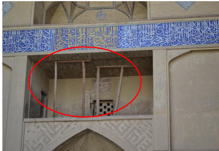
Fig 3.13. a) Use inappropriate scaffold to keep walls, arcs and other parts of mosque instead of repair them, b) Use inappropriate wooden and steel scaffolds to keep floors instead of use appropriate devices or repair techniques
