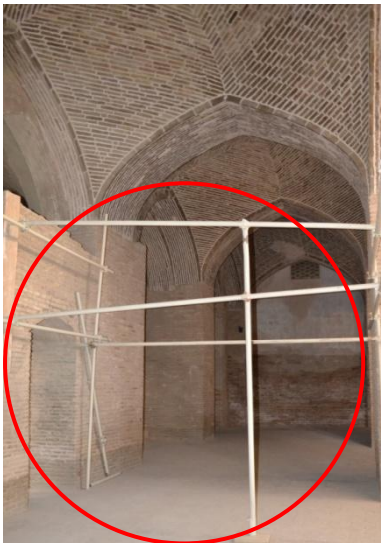
Fig 3.13. a) Use inappropriate scaffold to keep walls, arcs and other parts of mosque instead of repair them, b) Use inappropriate wooden and steel scaffolds to keep floors instead of use appropriate devices or repair techniques
