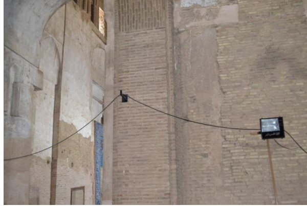
Fig 3.14. Using inappropriate hooks in the masonry walls of Masjed –e Jame without considering hook types and the thing is hanged in a) and b)
