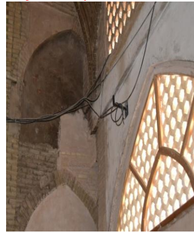
Fig 3.15. Both figures a and b are shown the unsuitable electrical wiring and lamps
