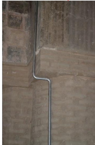
Fig 3.17. Unsuitable gas piping, both Figures a and b are shown the available inappropriate gas pipes before and after registration in UNESCO list
