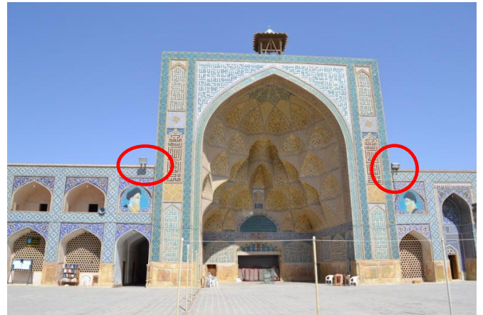
Fig 3.21. Photographs a and b are shown unsuitable external lights projecting from building
