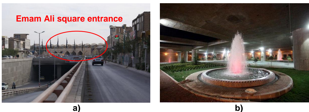
Fig 3.6. Completed underground highway (approximate date 2012), a) High way entrance and Emam Ali square entrance; b) Under the high way tunnel [51]
