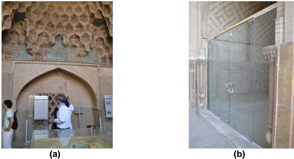
Fig 2.9. Visitor's Information Area adjacent to East Entrance. (Sep. 2013, by author) a) Inside the visitor information area; b) Glass door separated the visitor area from the passage way to the courtyard
