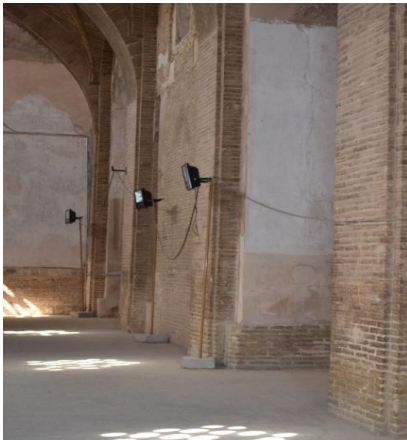
Fig 3.15. Both figures a and b are shown the unsuitable electrical wiring and lamps
