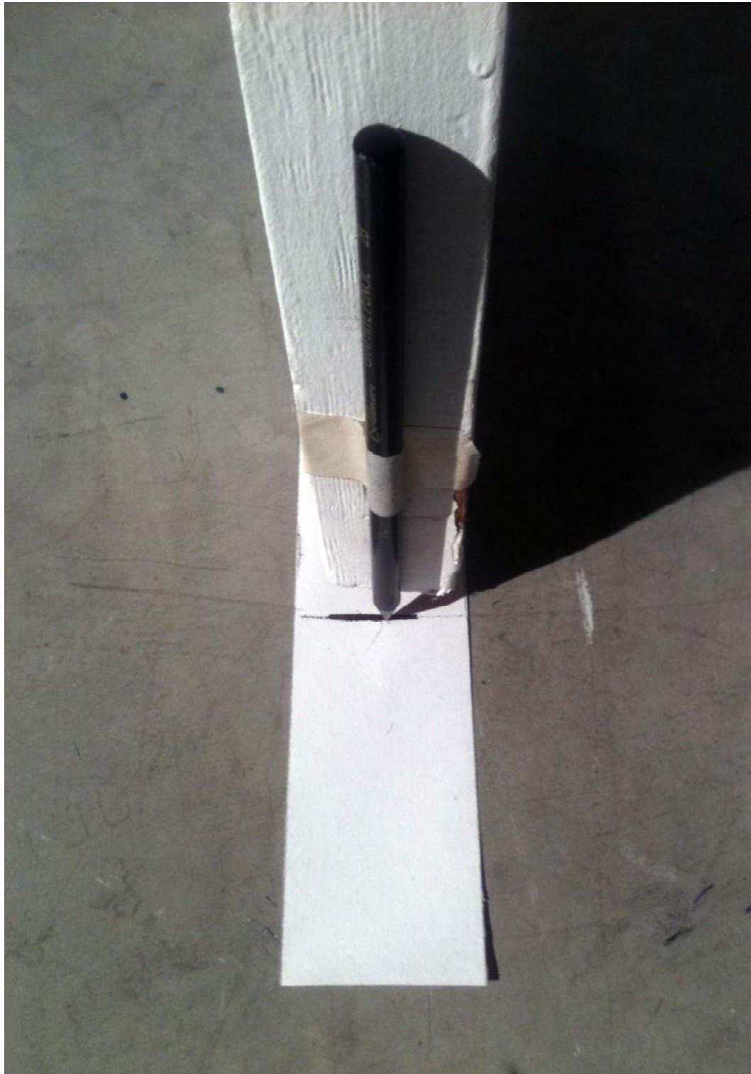
Figure twenty: Door One
