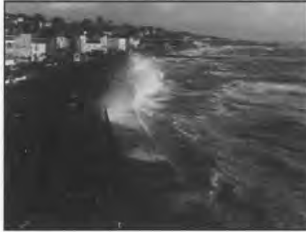
Figure 1.6: Image showing overtopping of the Dawlish seawall with potential flooding of the train line.
