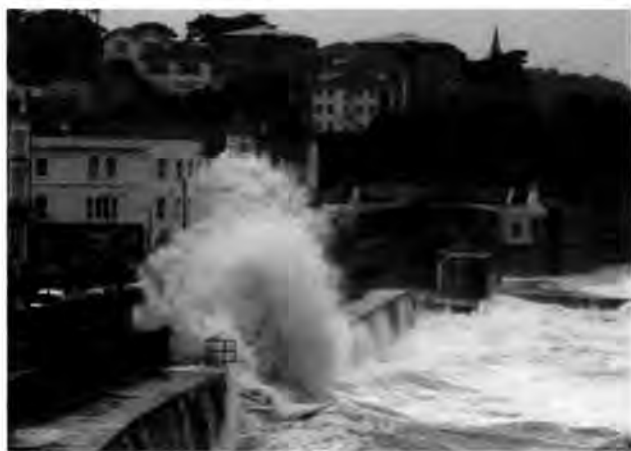
Figure 1.4: Image showing extreme waves impacting and overtopping the Dawlish seawall and flooding the train line.
