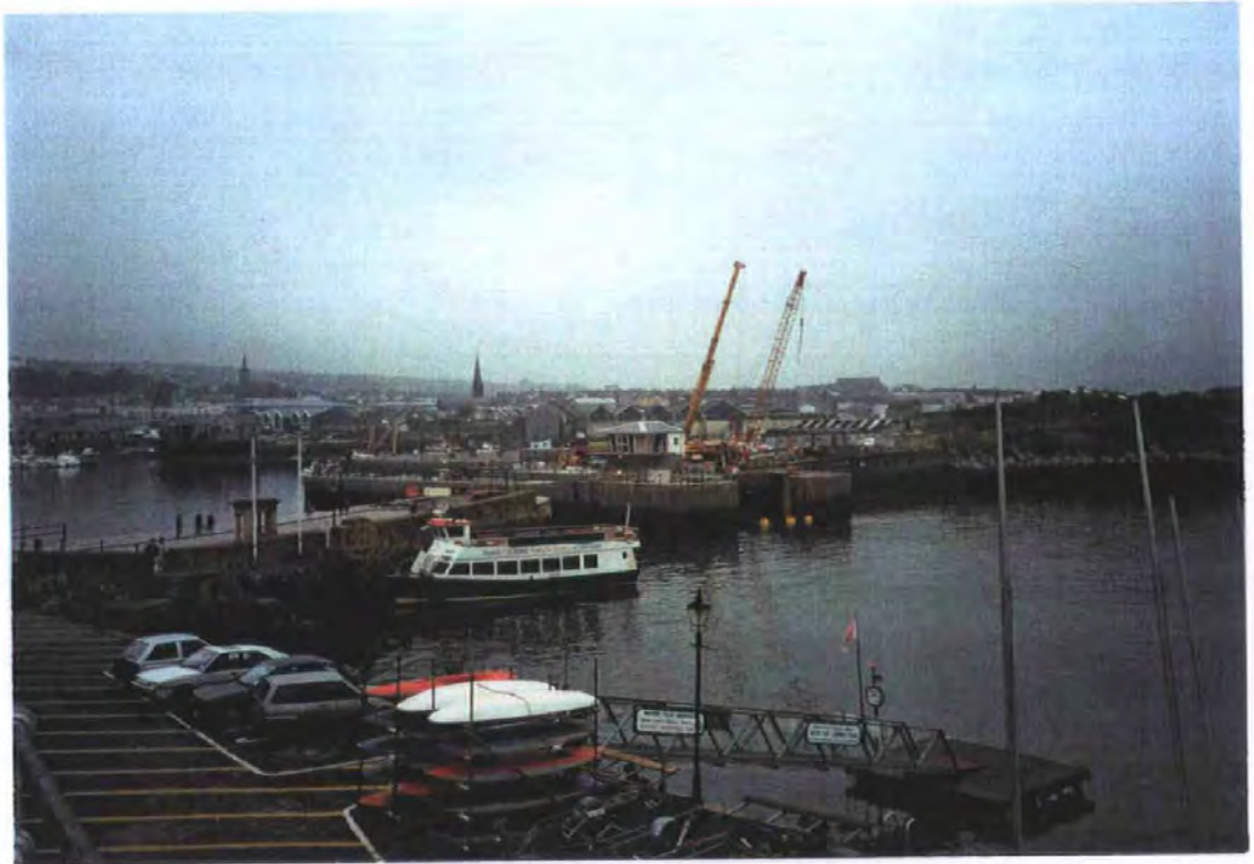
Plate 1.4. View to the north east overlooking the harbour mouth with the lock chamber (centre) in its final position. The control room can be seen and the scheme is in the final stages of completion. Note the restricted temporary harbour entrance (behind vessel) before the removable stop-log gate was positioned.
