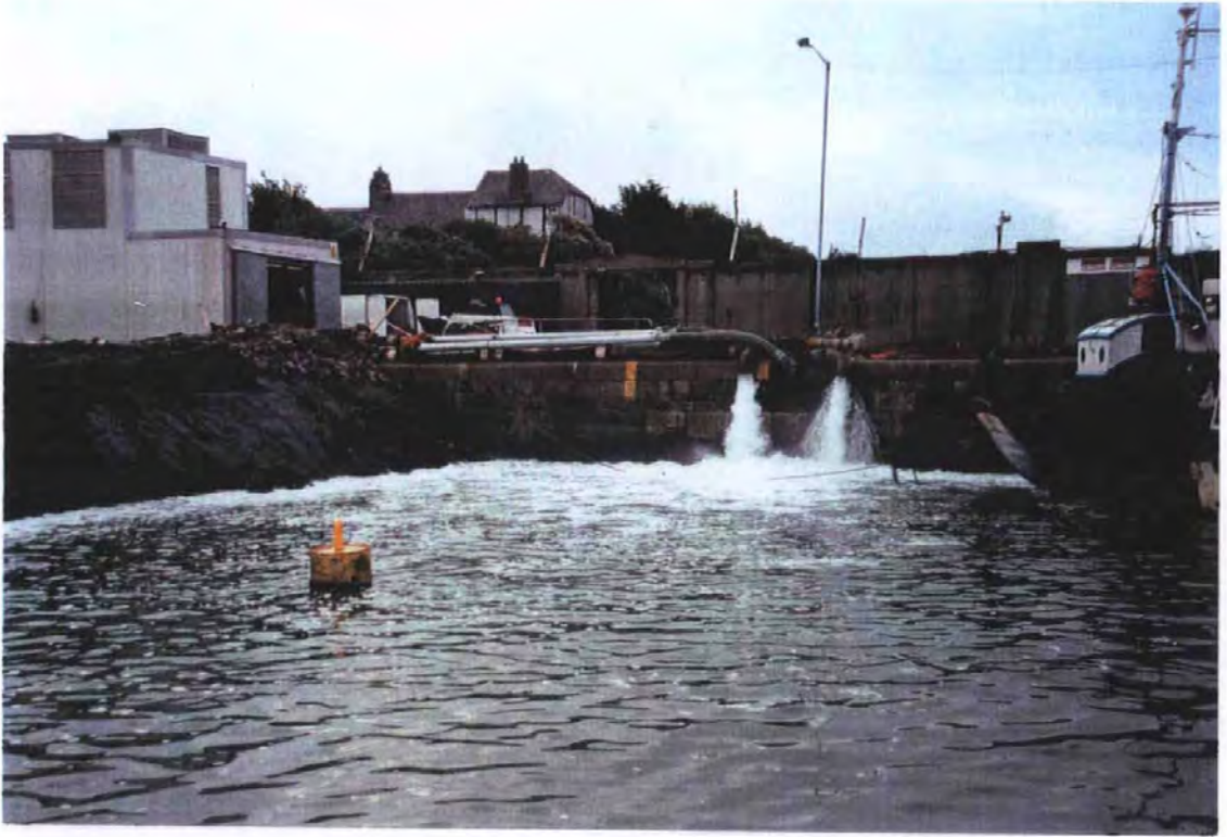
Plate 1.3. View to the south in the eastern arm of the harbour showing the clay-cored coffer dam (left) and the extensive pumping of water from behind the coffer dam into the main harbour to maintain the dry dock.
