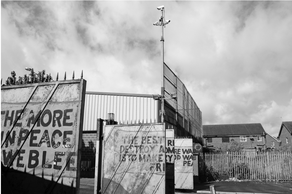
Figure 13.1 The condition of the Falls-Shankill 'peace line' at the Lanark Way gates, Belfast. Photograph by James O'Leary (2020).
