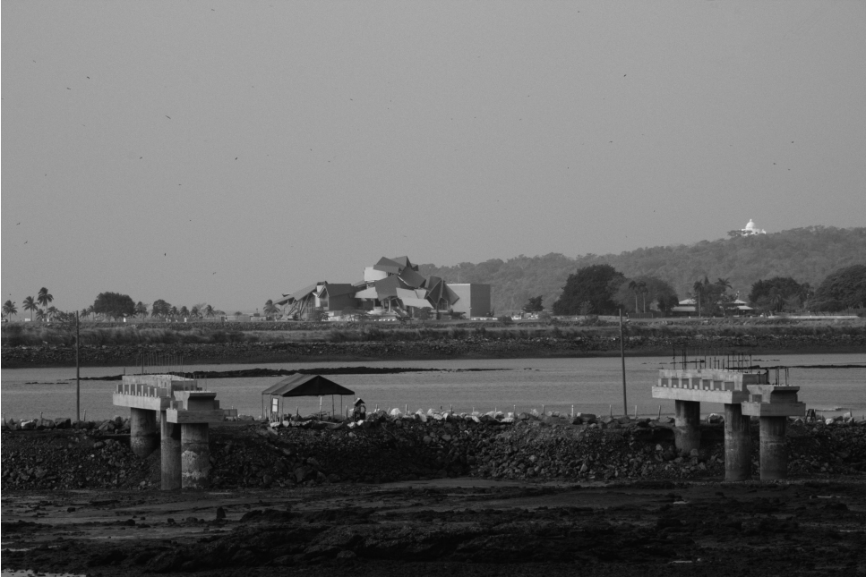
Figure 28.4 Construction of the Biomuseo from the viewpoint of la Plaza de Francia. Architect: Frank O. Gehry. Photograph by Ayaita (2013). Creative Commons Attribution-Share Alike 3.0 Unported. No changes made to image; no endorsement implied by use of this work.
