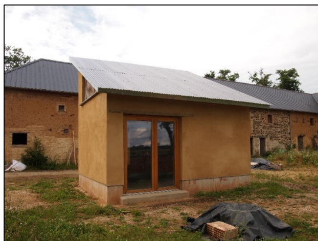
Figure 2. Global view of the CobBauge prototype building.
