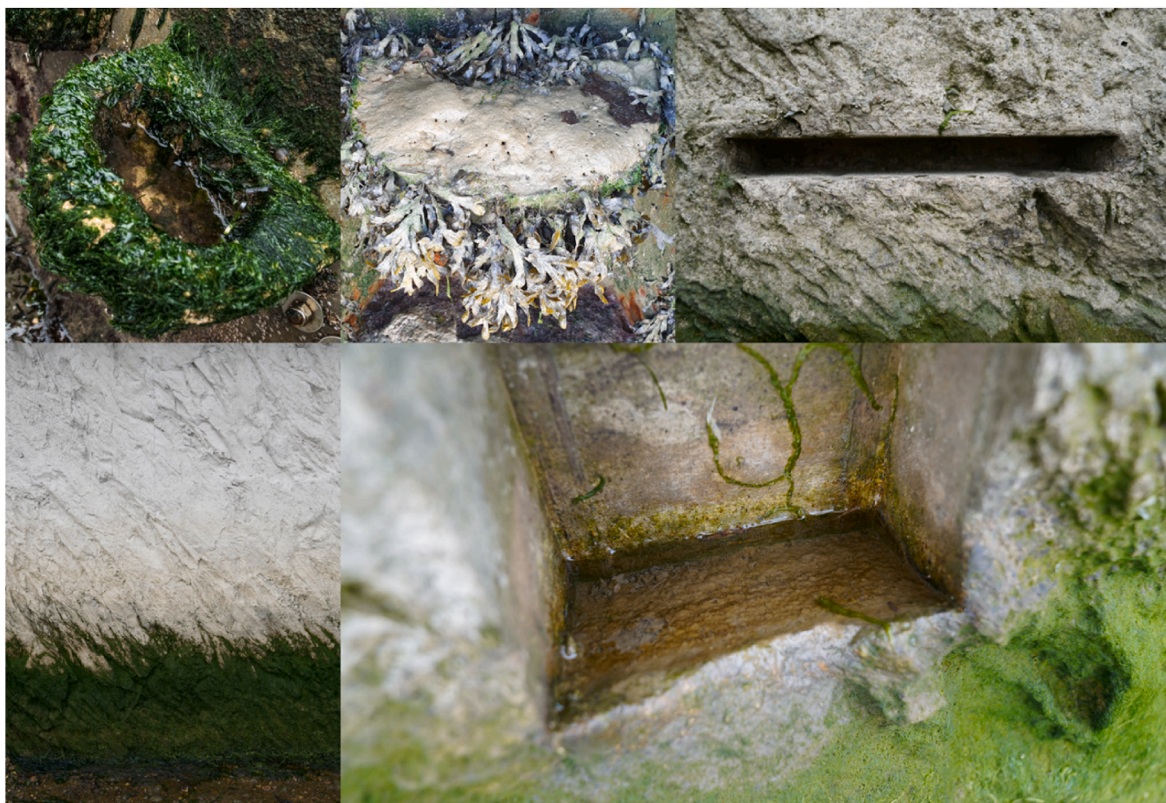
Fig. 2. Examples of coastal eco-engineering. Top left, clockwise: An artificial rockpool containing water (Marineff Project); a Vertipool containing mud (Bone et al., 2022); a ‘letter box’ crevice in a concrete seawall; a cubic void containing water in a concrete seawall; a concrete seawall with a ‘rockface’ textured surface created with a formliner. Images by Jessica R. Bone.
