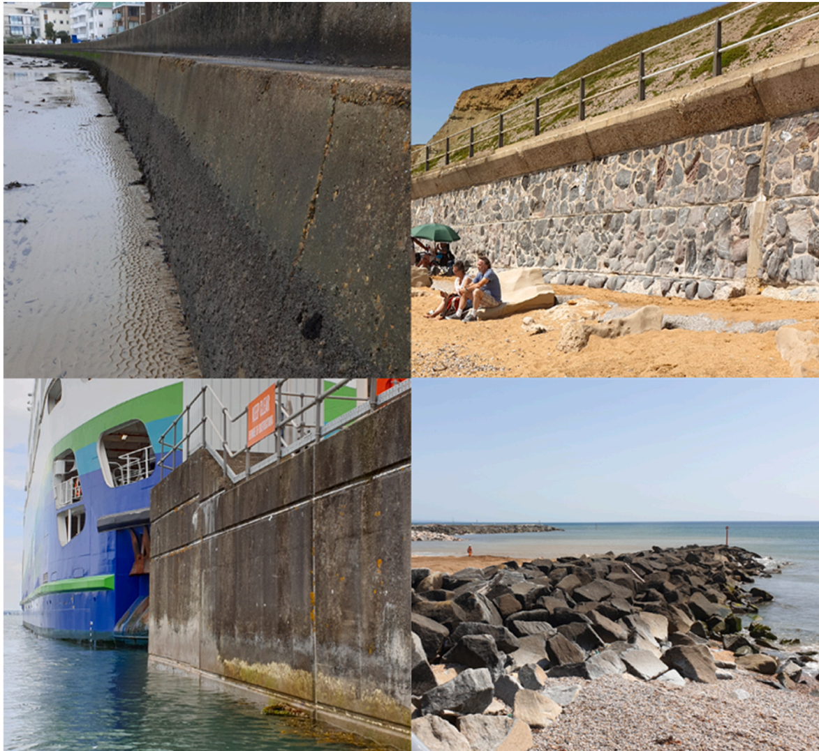
Fig. 1. Examples of artificial coastal structures (ACSs). Top left, clockwise; a concrete seawall; a stone masonry seawall; a rock groyne; concrete dock. Images by Jessica R. Bone.
