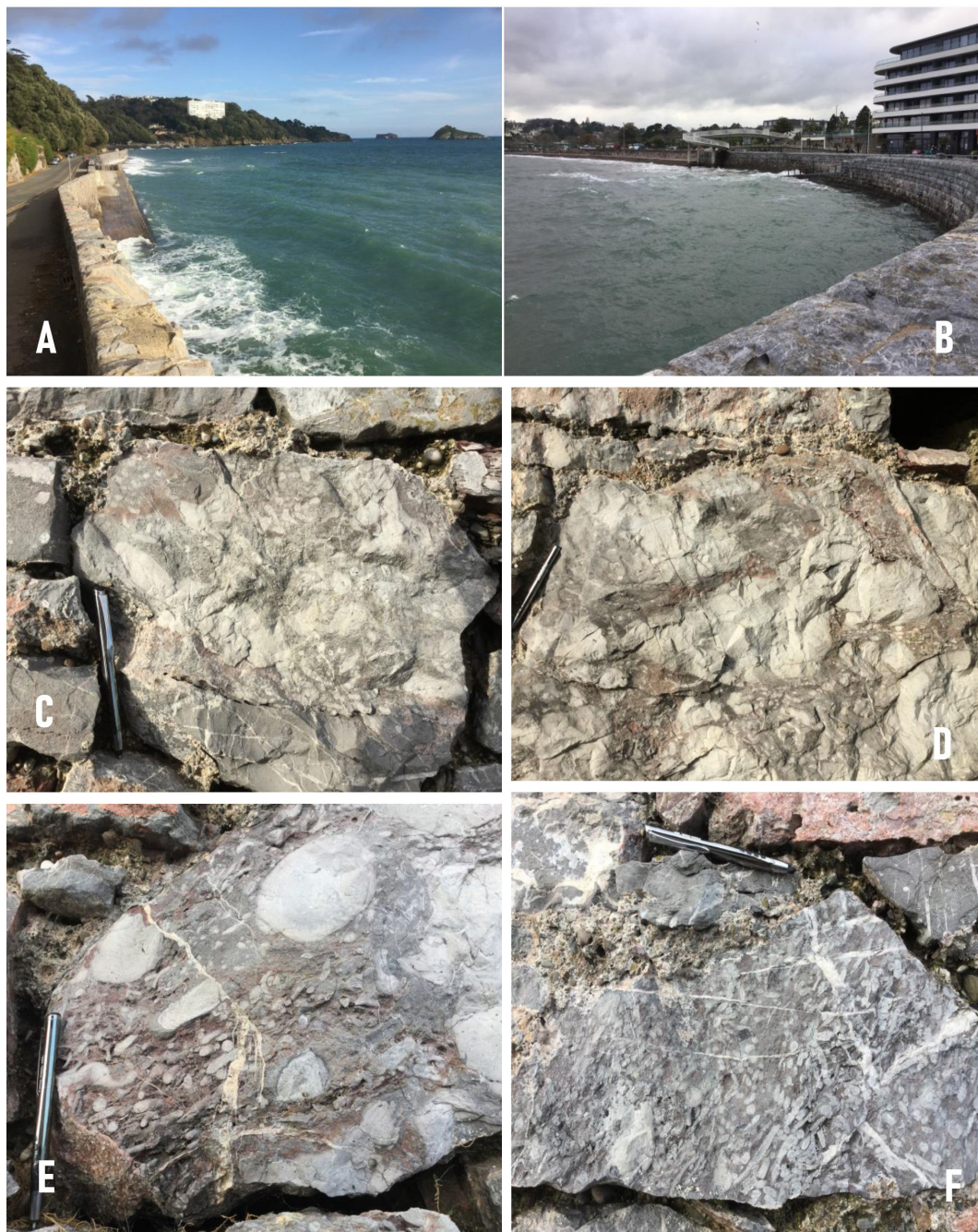
Figure 14. Promenade walls in A) Meadfoot Beach (with Kilmorie Flats, Ore Stone [flat top] and Thatcher Rock [pointed top] in the distance, B) Adjacent to Torre Abbey Sands. Inspection of these blocks of the Torquay Limestone Formation allow the identification of both the coral assemblages (tabulate and rugose) and the stromatoporoids (Fig. 14C-F). Note the 13 cm long pen for scale.
