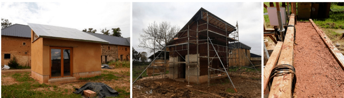
Figure 3. View of the prototype building and the in situ implemented instrumentation.
