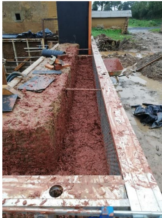
Figure 1. In situ implementation of a CobBauge double walling system.
