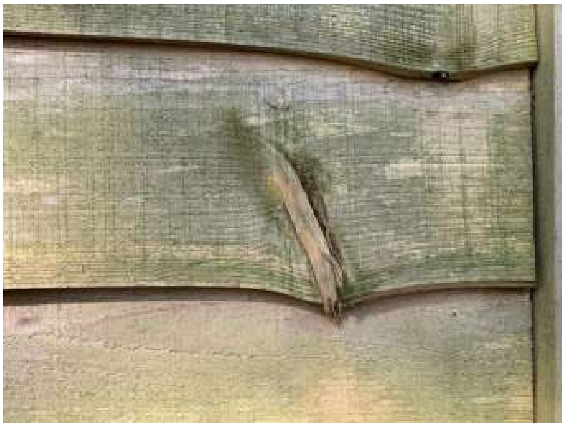
Figure 16: Plank section showing raised feature in in knot.
