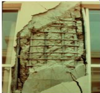
Damage class IV: Exposed rebars without buckling or fracture
