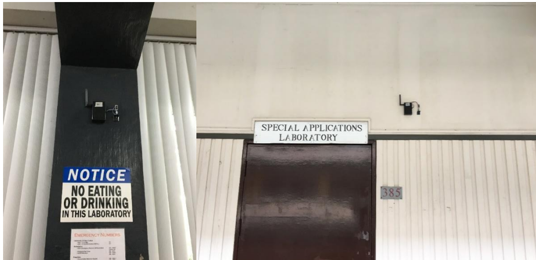
Figure 5.8 Sensors in position at different locations at USC, Cebu, Philippines (Source: Rabuya, 2017).
