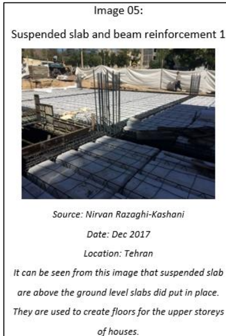
Figure 5.14 Images of suspended floor slab ready for concrete in Tehran, (source: Nirvan Razaghi-Kashani).
