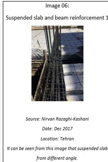
Figure 5.14 Images of suspended floor slab ready for concrete in Tehran, (source: Nirvan Razaghi-Kashani).
