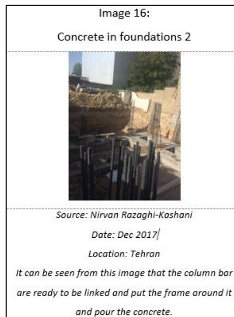
Figure 5.13 Images of finished concrete building foundations in Tehran, (source: Nirvan Razaghi-Kashani).
