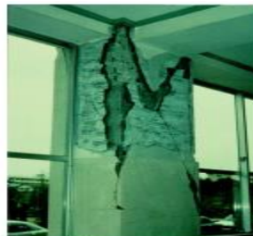
Damage class III: (left) Cracks with a width of about 2mm on structural concrete (right) Spalling concrete cover and slightly exposed rebars
