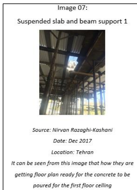
Figure 5.15 Images of support to suspended floor in Tehran, source (Nirvan Razaghi-Kashani).
