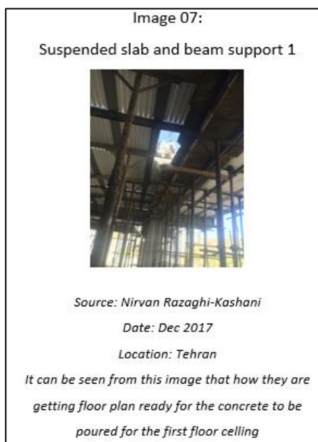
Figure 5.15 Images of support to suspended floor in Tehran, source (Nirvan Razaghi-Kashani).
