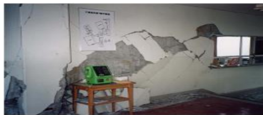
Damage class IV: Exposed rebars without buckling or fracture
