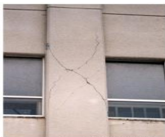
Damage class III: (left) Cracks with a width of about 2mm on structural concrete (right) Spalling concrete cover and slightly exposed rebars
