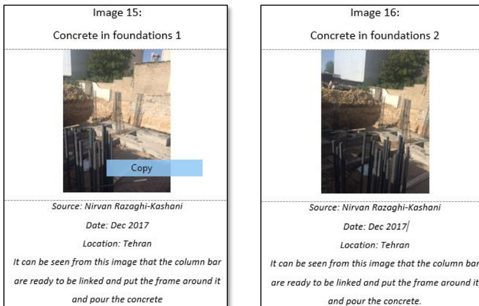
Figure 5.13 Images of finished concrete building foundations in Tehran, (source: Nirvan Razaghi-Kashani).
