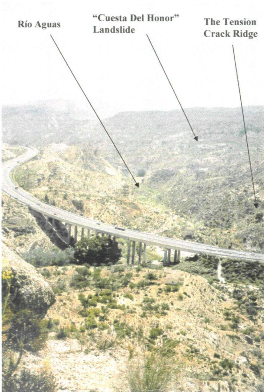
Figure 5.41 – Photograph of the elevated section of the E-15 Motorway above the Río Aguas (Grid Reference: 0583041055 / Facing east).
