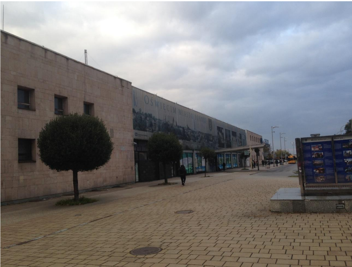
Figure 5 Oświęcim railway station, 2018
