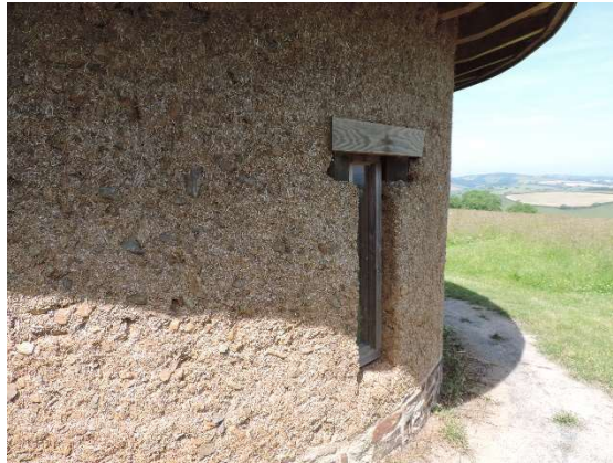
Figure 1. Exposed cob construction in Totnes, UK.
