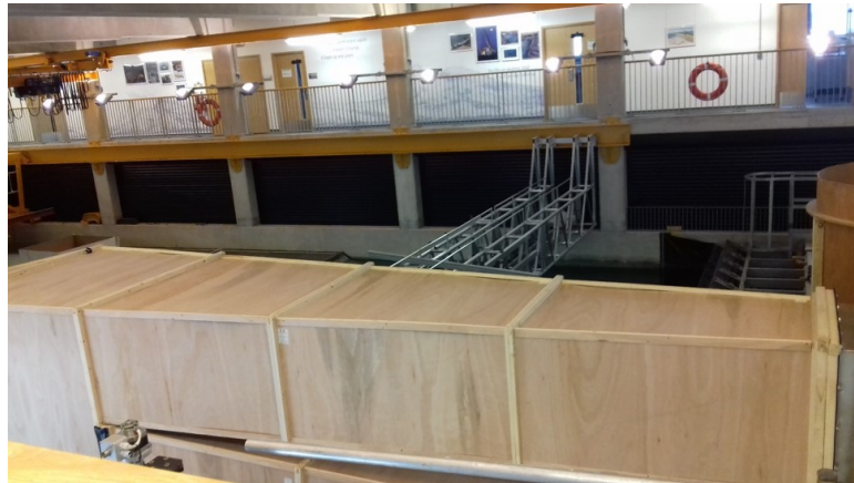
Figure 5.30: Wooden structure to combine the airflow of the two fans
