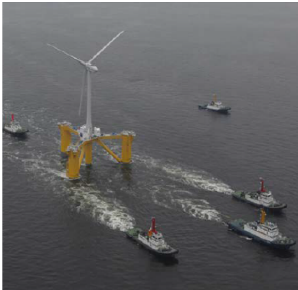
Figure 2.10: Towed Fukushima Mirai wind turbine. Photo taken from Ishihara et al. (2014) with permission of T. Ishihara. Original photo: Photo of the WindFloat 2 MW prototype installed in 2011 near Portugal. Ballasting and connection to the offshore tug vessel Bourbon Liberty 228 (Principle Power, 2011). Had to be taken out, as copyright owner could not be contacted
