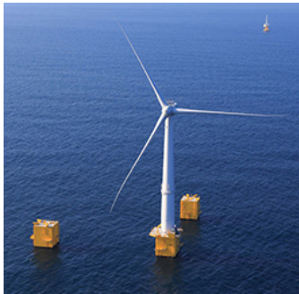
Figure 2.9: Fukushima Shinpu 7 MW wind turbine using V-shaped semi-submersible platform (taken from Sawaji (2016), also found in Fukushima Off-shore Wind Consortium (n.d.b), with the permission of T. Ishihara)
