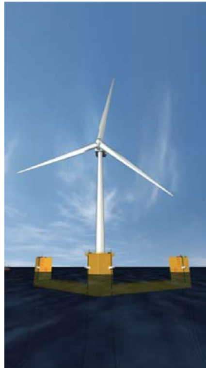
Figure 2.8: Fukushima Shinpu 7 MW wind turbine using V-shaped semi-submersible platform (taken from Ishihara et al. (2014) with the permission of T. Ishihara). Original image from PowerTechnology (n.d.) was taken out as copyright owner could not be contacted
