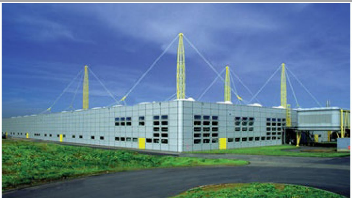
Figure 5.18 Igus factory showing interchangeable cladding units: Grimshaw Architects
