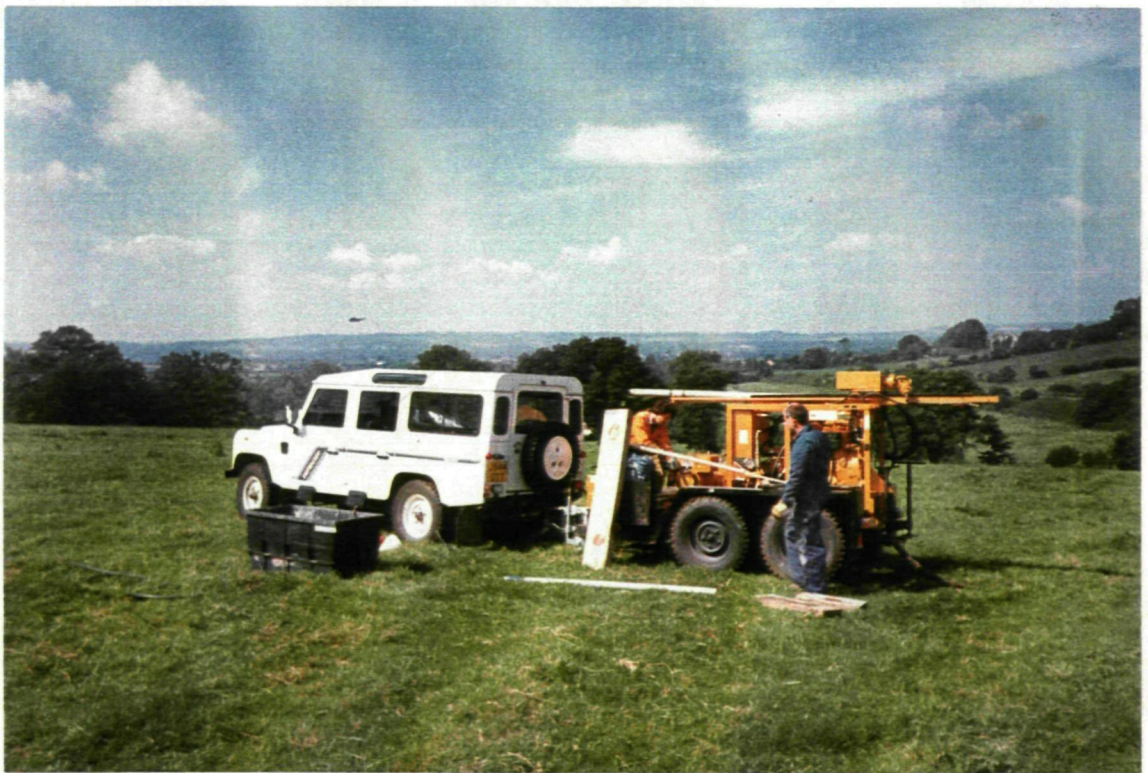
Figure 2.1. The B24 Mobile Surveyor Drilling Rig in operation on the site of the Hartmoor Hill Borehole, north Dorset.
