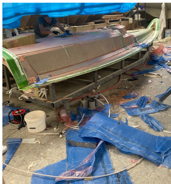
Fig. 2: Typical single use resin contaminated flow mesh with release film being stripped off cured part after each cycle
