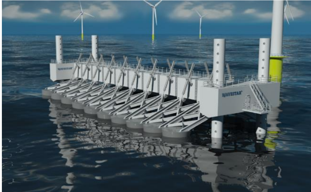
Figure 2.9: The Wavestar point absorber system [26].
