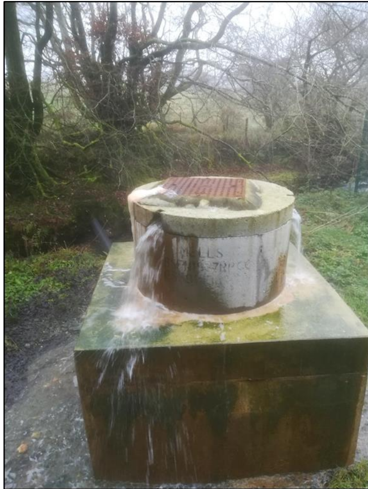
Figure 3.3 Outfall drain overflow at Inny Vale, November 2019
